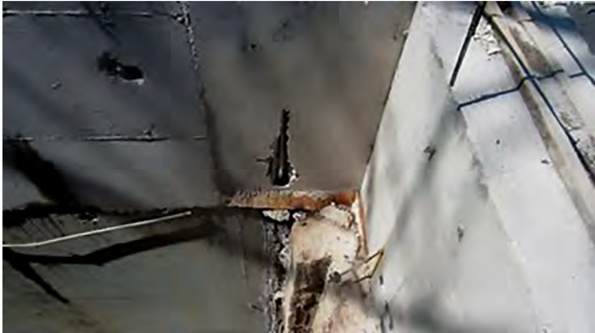
Inadequate covering of the rebars (Andriolo’s Archive)
