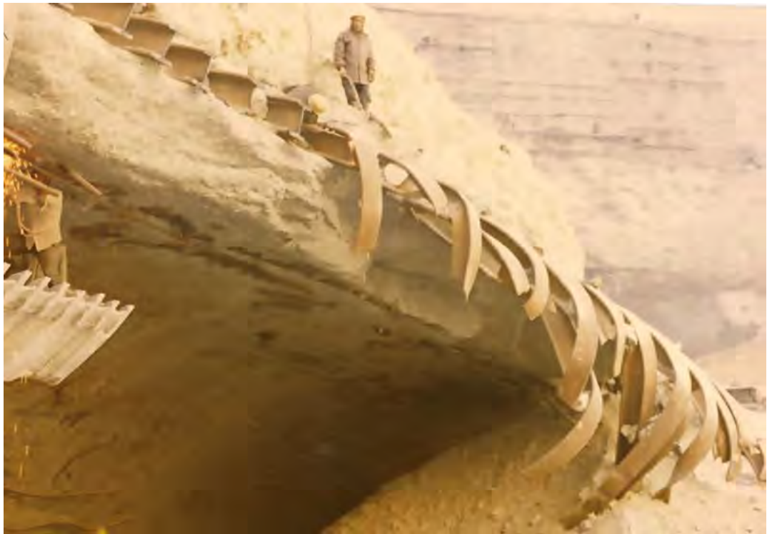
Tunnel 2 collapse, diameter 13,3 m and 6 inches steel ribs HEM 360 (courtesy R. Allione)
