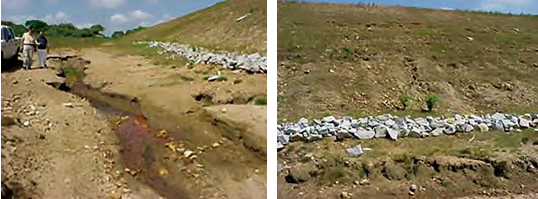
Figures showing sparse vegetation and erosion downstream of an embankment slope (Pictures from Andriolo's archives)
