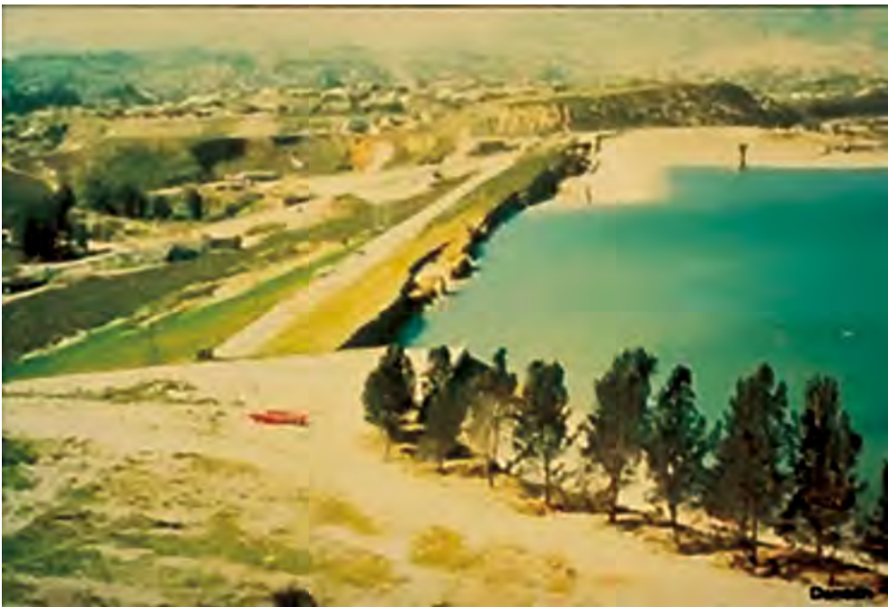
This aerial view shows how the crest of the dam disappeared under the reservoir as a result of the slide in the upstream shell. The slide occurred shortly after earthquake shaking ended and was attributed to loss of strength in the hydraulic fill due to liquefaction.
