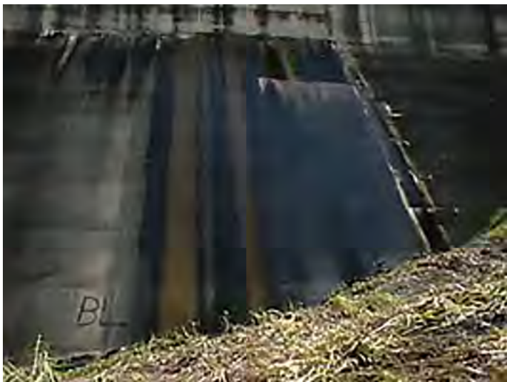
Poor quality of RCC in a dam due to inadequate construction joint surface treatment and/or inadequate water tightness system (Pictures from Andriolo’s archives)
