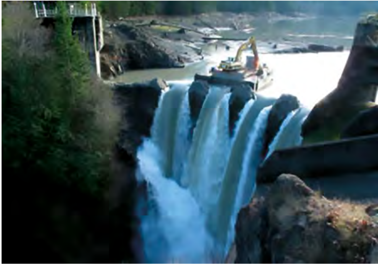
Demolition of Glines Canyon Dam by barge-mounted hoe ram that created a series of notches with which to drawdown the reservoir (Photograph courtesy of National Park Service)
