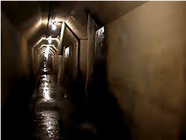
Poor quality of RCC in a dam due to inadequate water tightness system (Pictures from Andriolo's archives)
