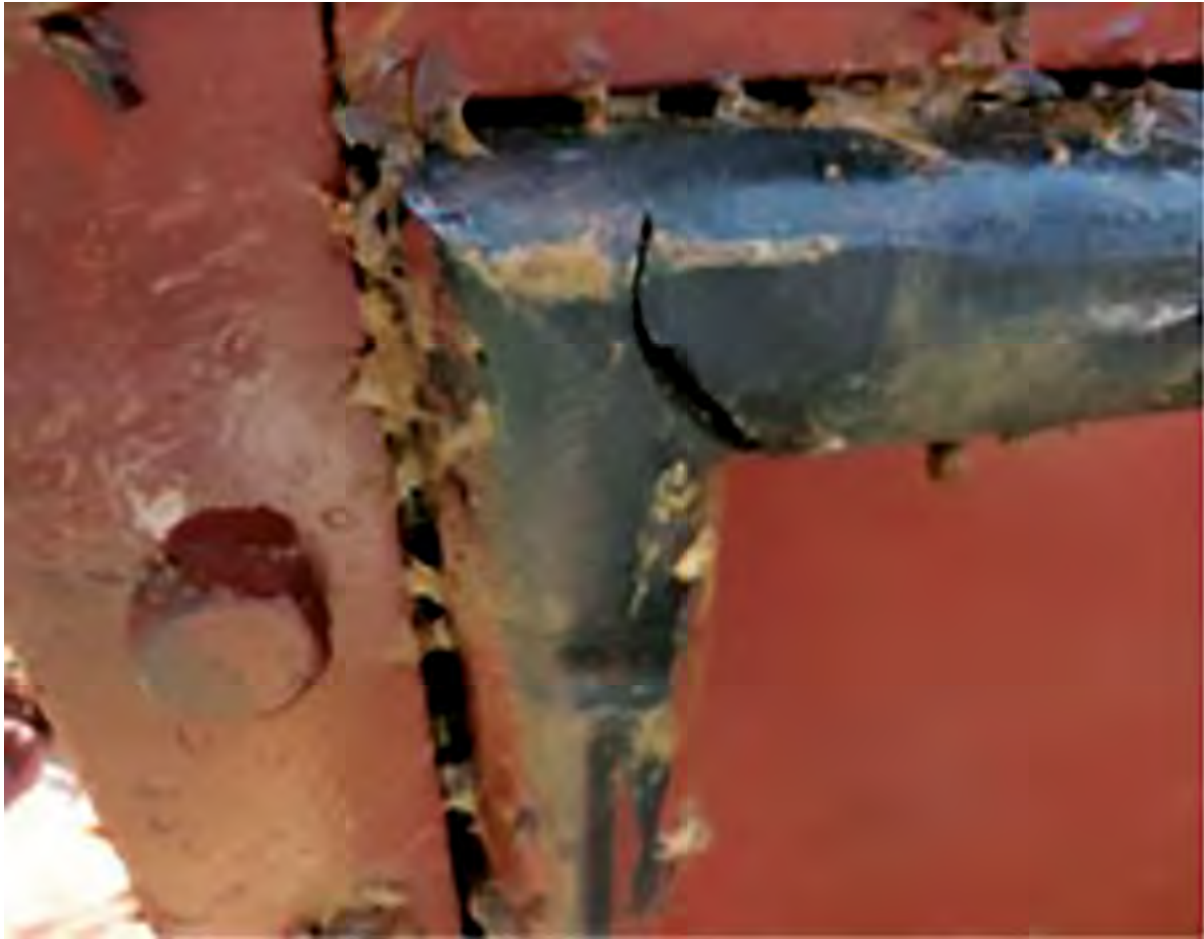
The rubber seal damaged
