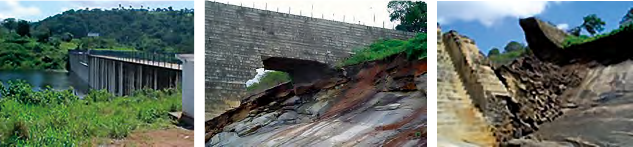
The Camará Dam as was constructed (at left above) and the damages due to the foundation collapse (Pictures from the Reference)
