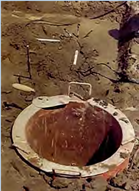
Sequence of installation of a strain meter spider and autogenous box in the mass concrete at Itaipu Project (From Andriolo's Archive, 1978)
