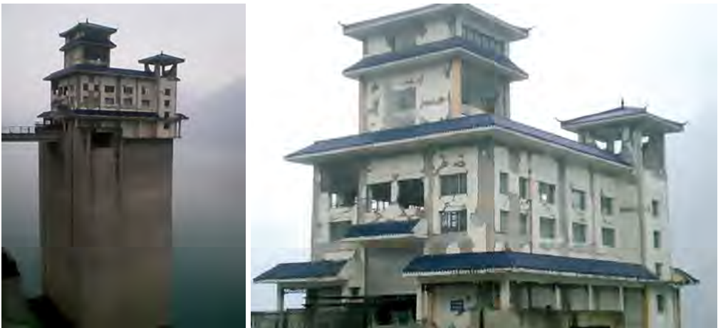
Damage of reinforced concrete building on top of the intake towers of the Zipingpu reservoir, after the May 12, 2008, Wenchuan earthquake [04-66]
