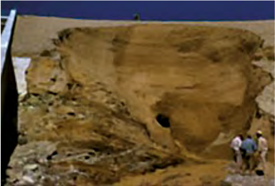
The erosion hole about noon on Saturday September 4. Note 1,2m-diameter leak exit tunnel adjacent to the right abutment rock.
