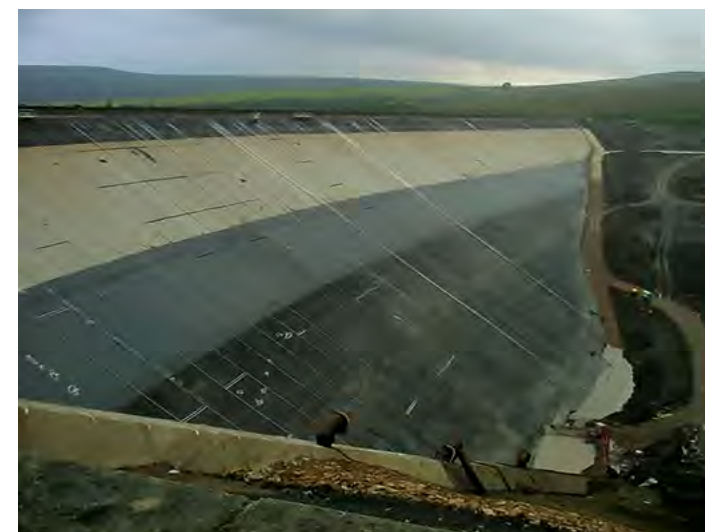
Back of Winscar Dam, Dunford Bridge. This dam started to leak in 2000 and was emptied so that it could be repaired.
