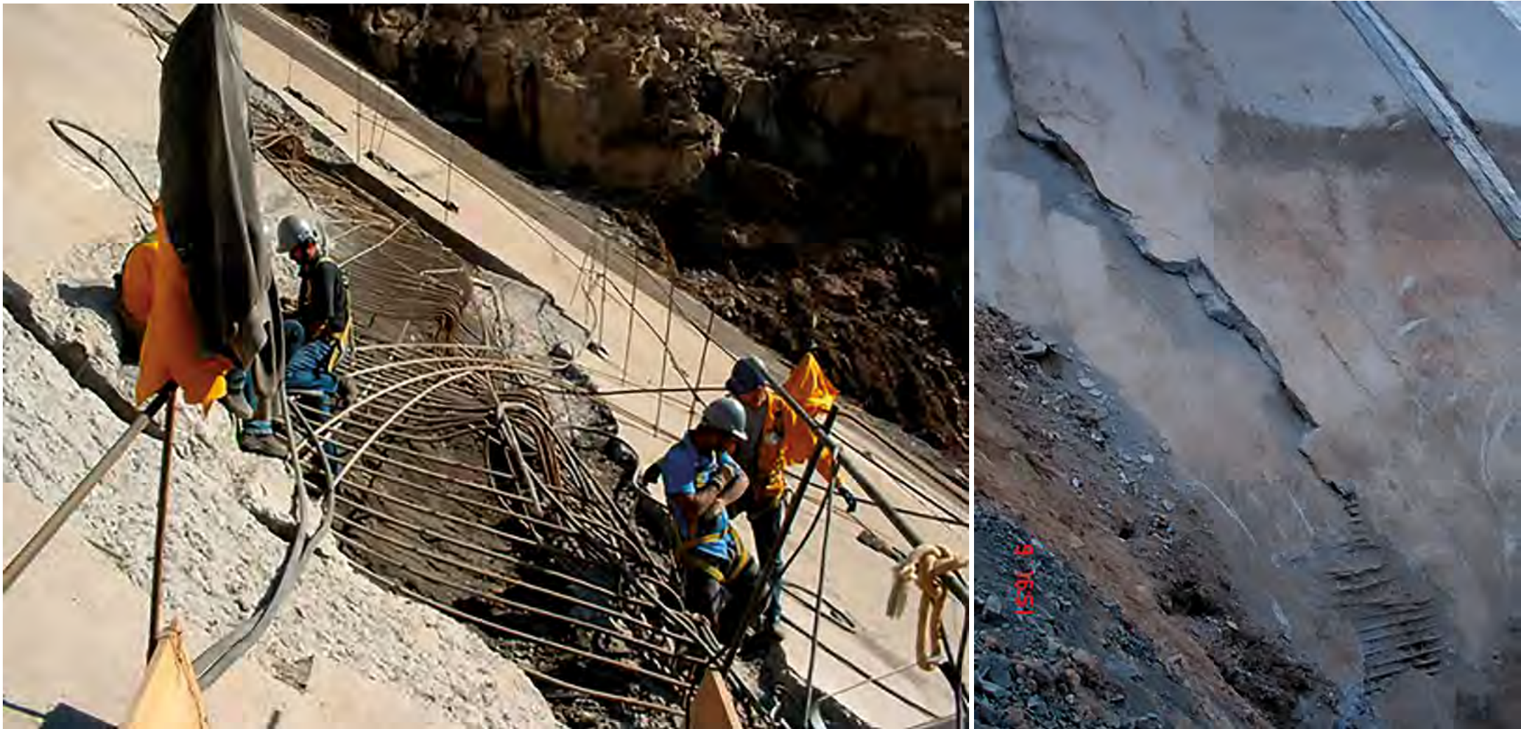
The damages at Campos Novos CFRD
