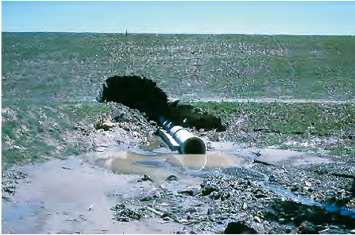
A failure due to internal erosion often leaves a tunnel-shaped void along the conduit [04-08]
