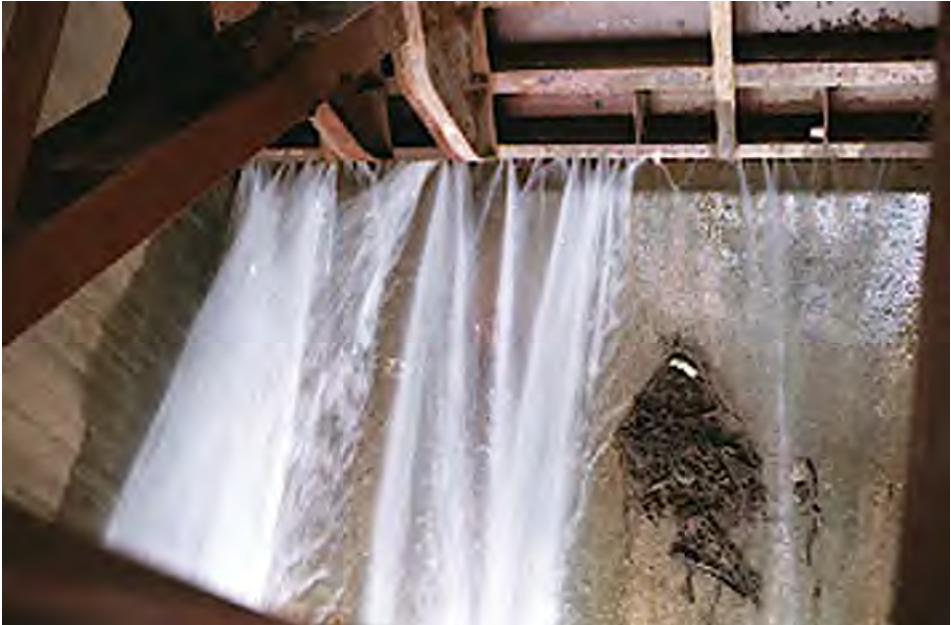
Damage of the radial gate of intermediate level spillway of Sefidrud dam caused by June 21, 1990, Manjil earthquake, large hydrodynamic pressures caused inelastic buckling of gate arms, gate distortions and leakage
