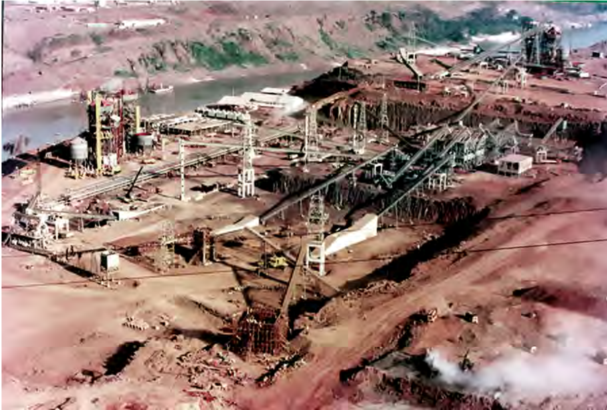
View of the assembling of the installations for the Production of Aggregate Material and Concrete Plants on the right bank of Parana River in April 1978
