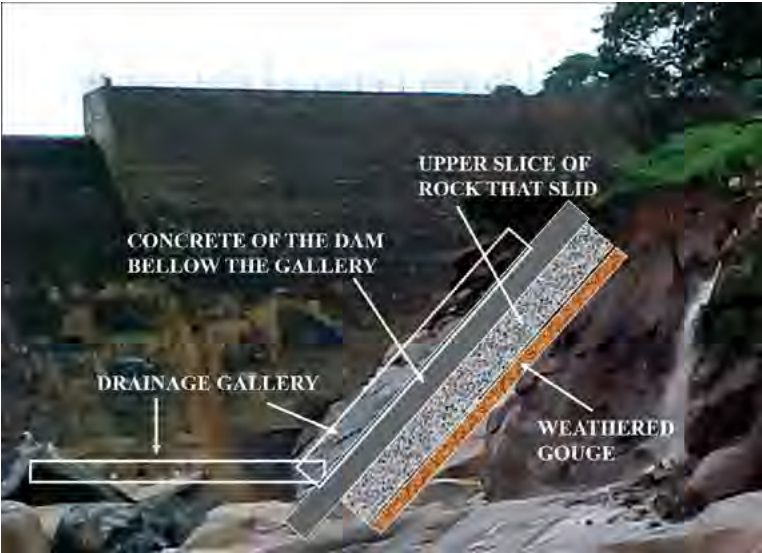
The Camará Dam as was constructed (at left above) and the damages due to the foundation collapse (Pictures from the Reference)
