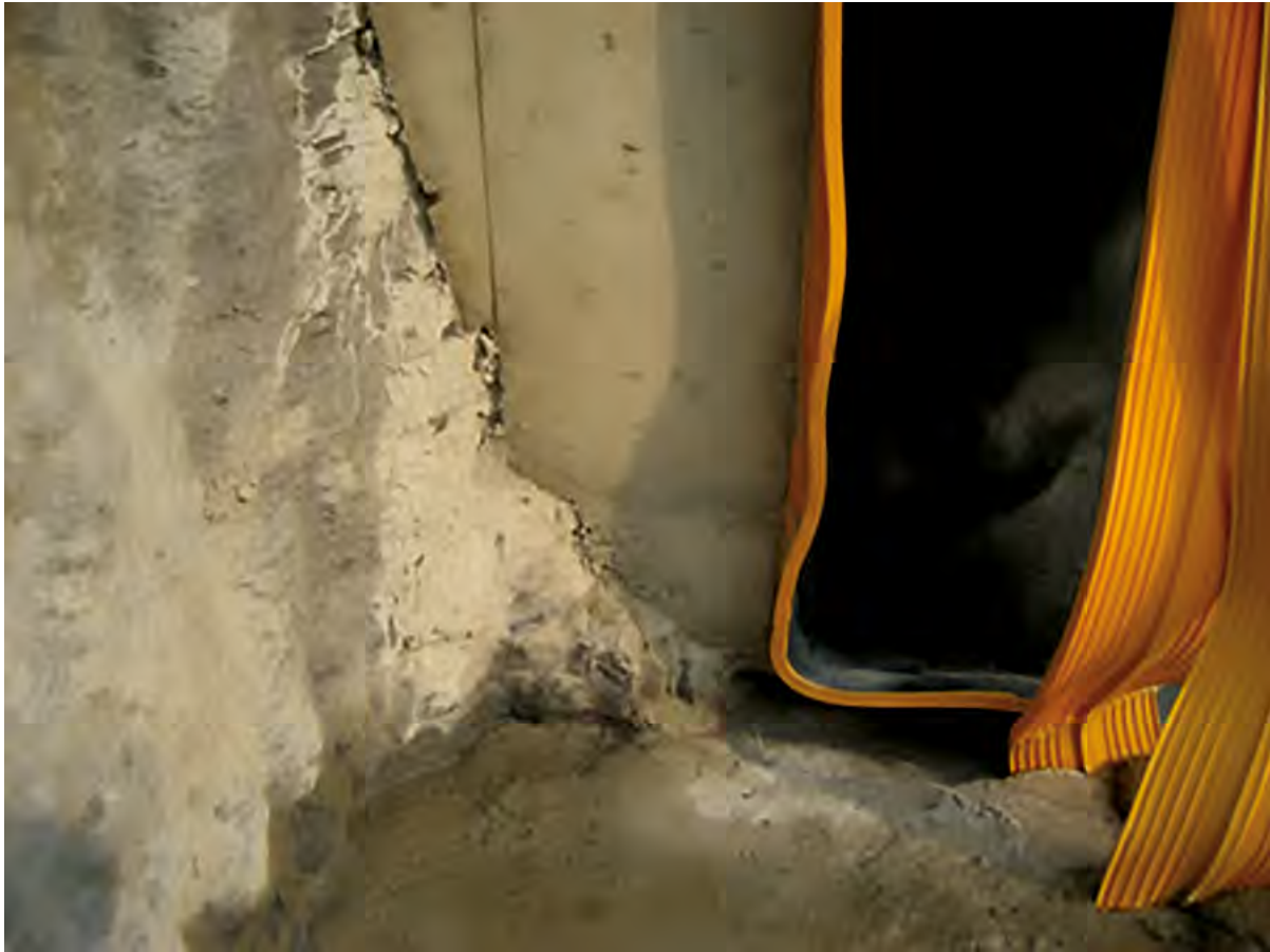
Lines of a PVC Waterstop near a rock foundation and an interface with a PVC membrane at Beidag RCC Dam - 2006 (Andriolo's Archive)
