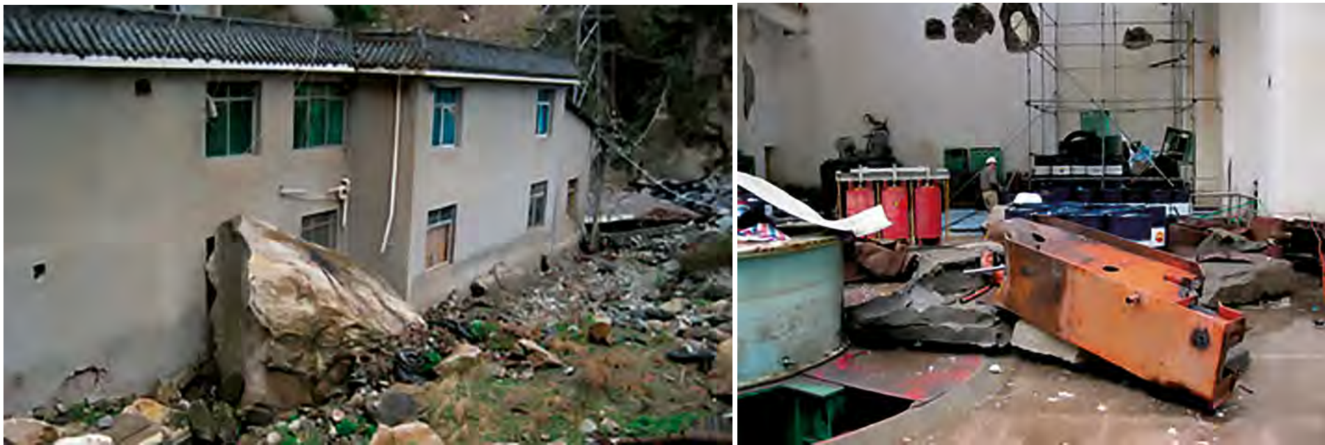
Damages in Shapai Powerhouse after the May 12, 2008 Wenchuan earthquake [04-66]
