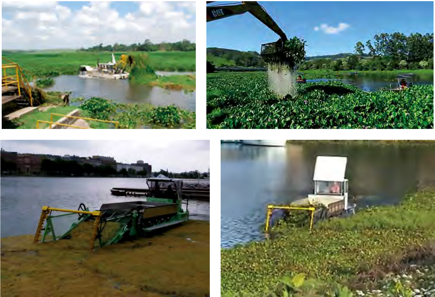
Pictures showing the removal of vegetation from a reservoir (from Ref. [09-09]).
