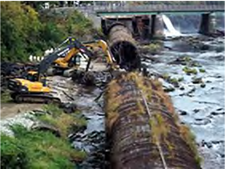
Penstock being replaced in Pepperell Dam
