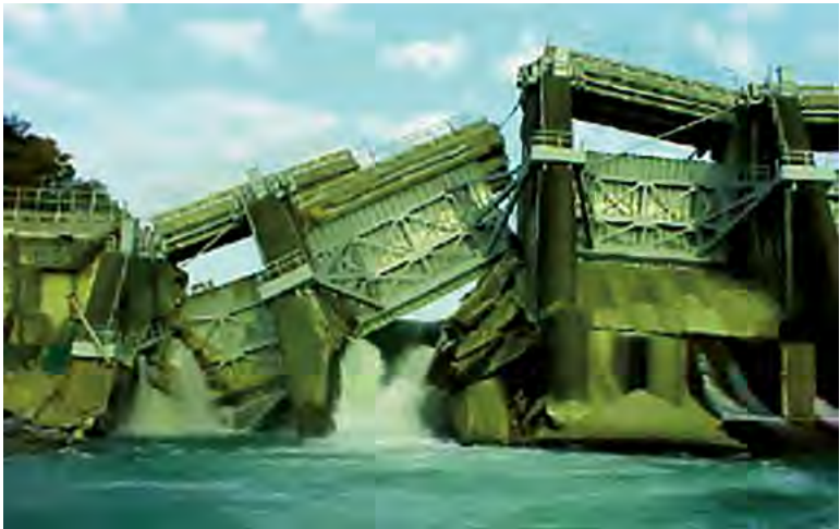
The damage caused by earthquake in the Spillway Shih-Kang Dam
