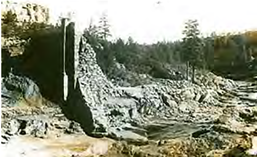
Castlewood Canyon Dam after the rupture (from internet)
