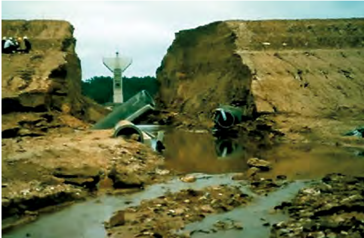
Failure of an embankment dam due to the discontinuity represented by the conduit [04-08]
