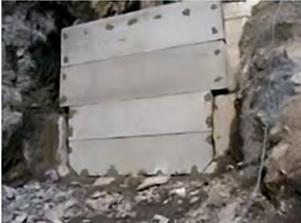
At Glines Canyon Dam, Washington, the upstream tunnel barrier (left) was blocked using precast concrete panels while the downstream tunnel barrier (right) was blocked using metal panels (photograph courtesy of Tom Hepler, Bureau of Reclamation.)
