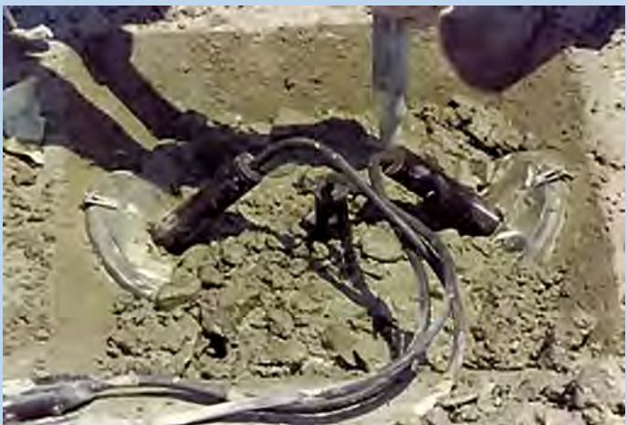
Sequence of installation of a stress meter set in the mass concrete at Itaipu Project (From Andriolo's Archive, 1978)
