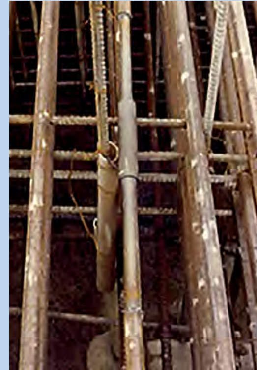
Installation of a reinforced meter in a reinforced concrete at the Itaipu Power House (From Andriolo's Archive, 1980)
