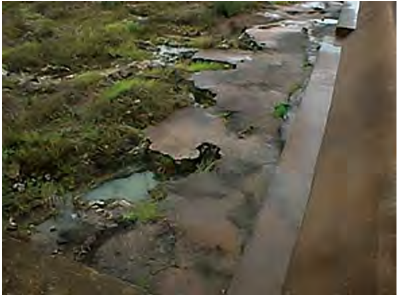
Concrete erosion on spillway surface due to poor concrete quality and lack of maintenance (Pictures from Andriolo's archives)
