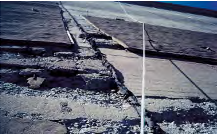
Views of the damages of the concrete face on Salt Springs Dam and the repair using a PVC Membrane
