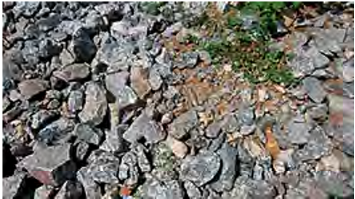
Details of poor riprap protection for the downstream slope of an embankment dam (pictures from Andriolo’s archives)
