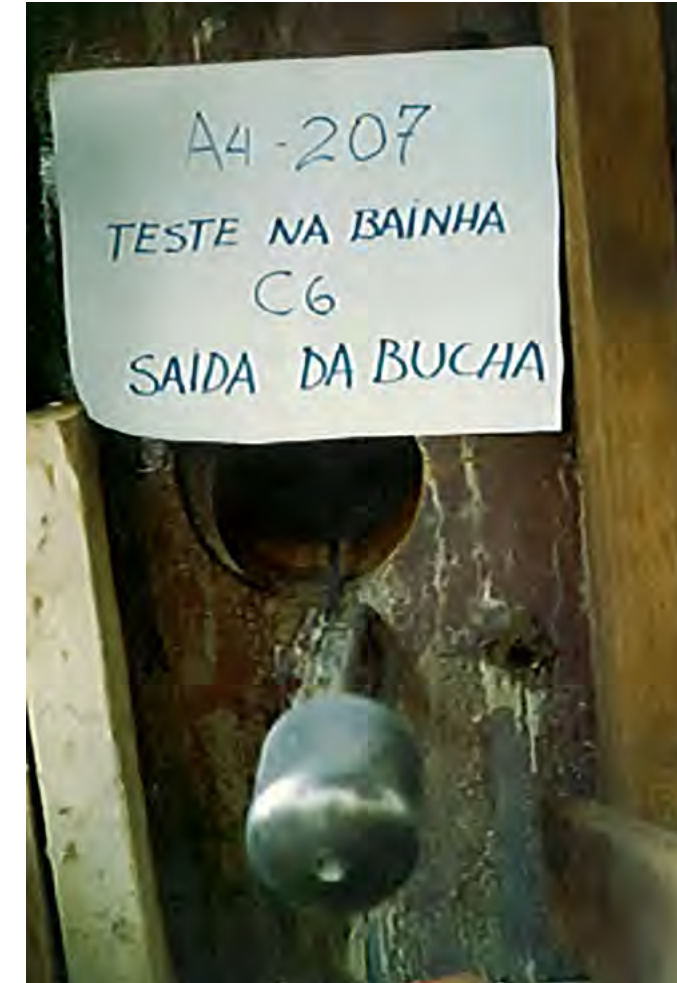
Ducts and tendons for post-tensioning a pier - Itaipu Spillway Piers - 1979 (Andriolo's Archive) [03-01]
