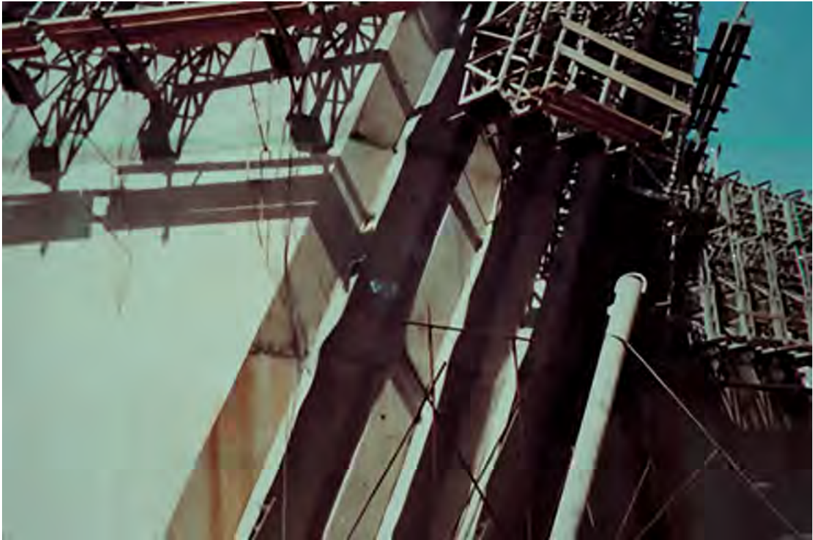
Three Lines of a PVC Waterstop - Itaipu Main Dam - 1979 (Andriolo's Archive)
