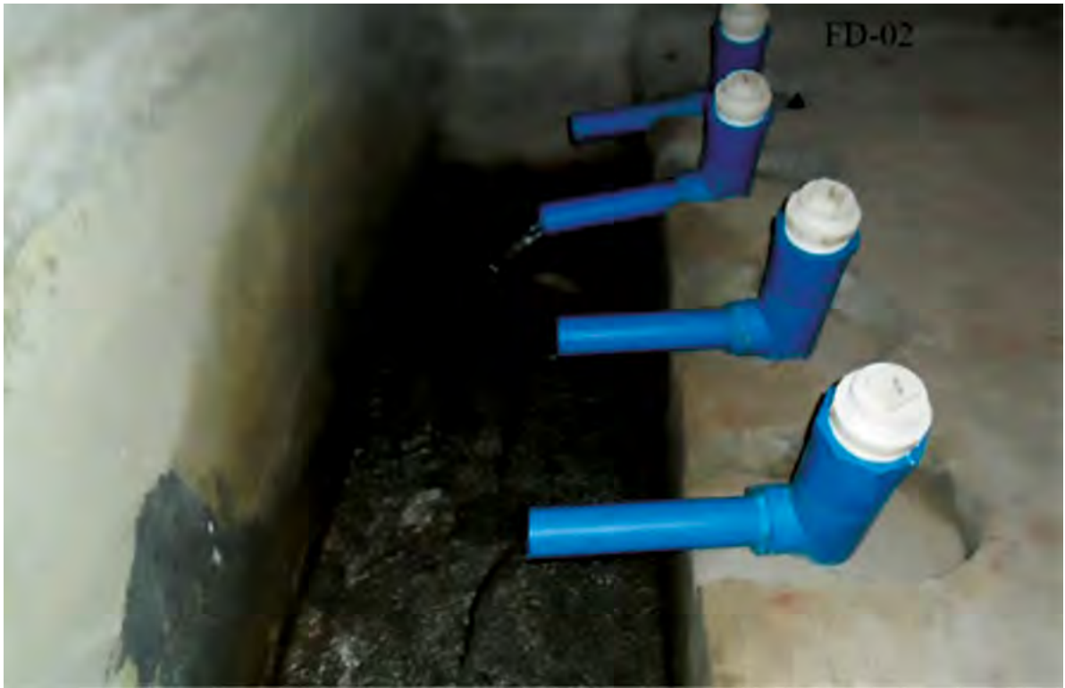
A satisfactory drainage system foundation (Pictures from Andriolo's archives)
