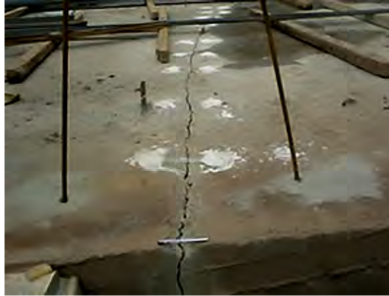
Thermal cracks observed in different concrete structures (Andriolo's Archive)
