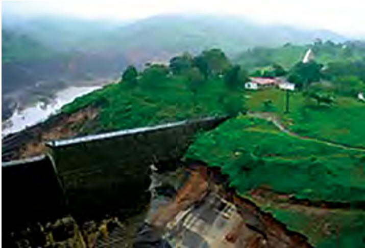
Camará Dam after failure (*)
