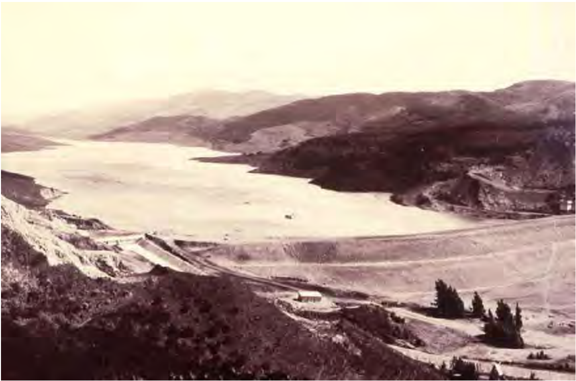
The San Pablo Dam near Oakland, California was a hydraulic fill embankment 67 m high, constructed in 1918-20. Buttress fill zones were placed up and downstream of the original dam in 1967 and 1979-80 to increase seismic stability.
