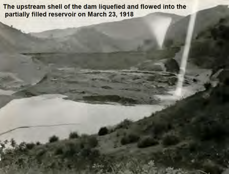
On March 23, 1918, the fill slid upstream in five minutes, destroying the intake tower
