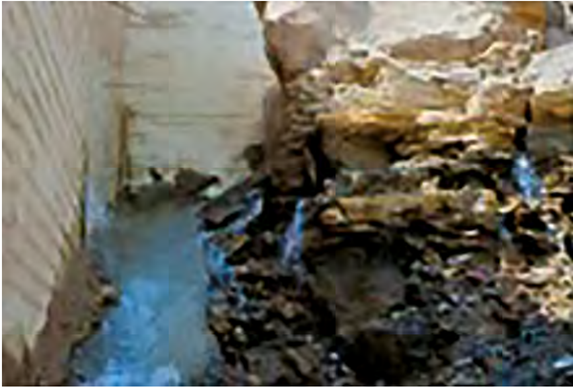
Third embankment slide. Seeps issuing from vertical cracks in sandstone.
