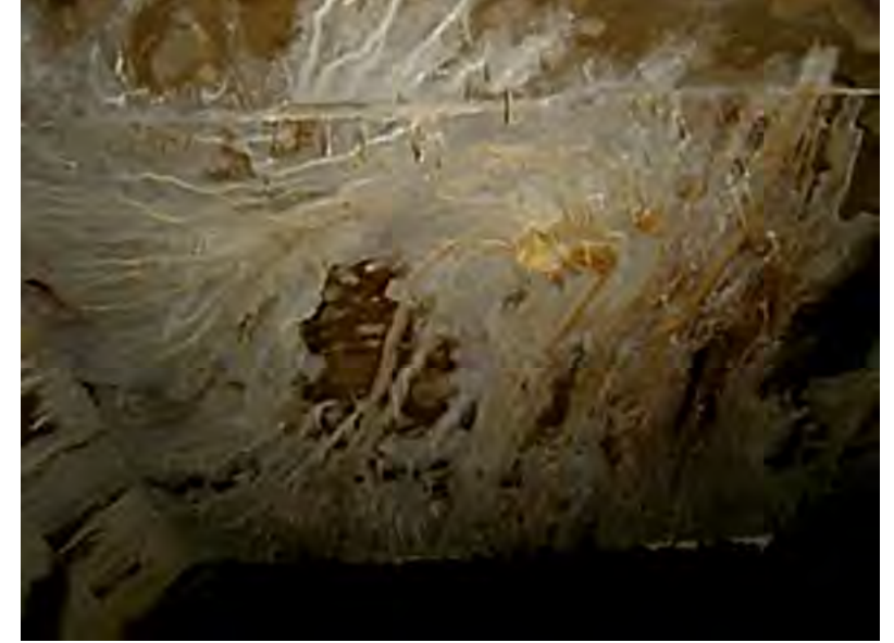
Leaching observed in the downstream face of a Dam and in the inner part of the dam gallery-(Andriolo's archive)
