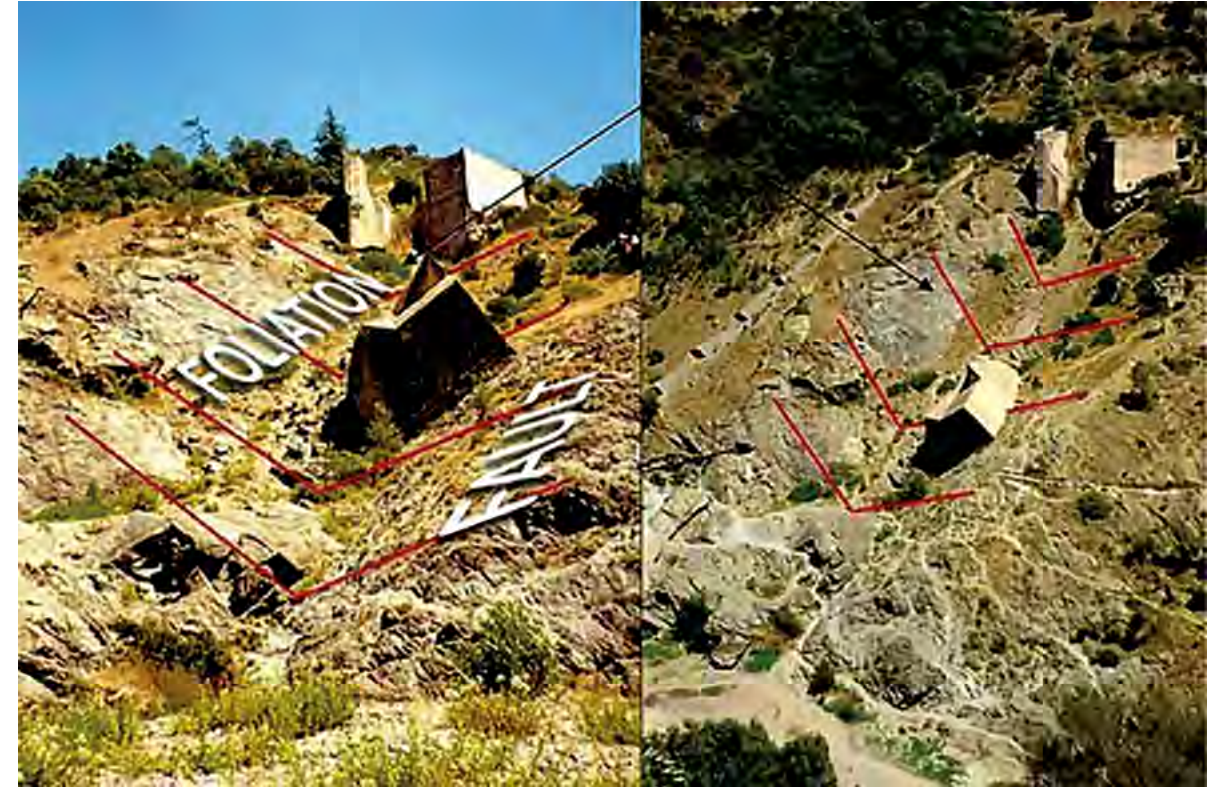
Malpasset failure surfaces seen from the ground
