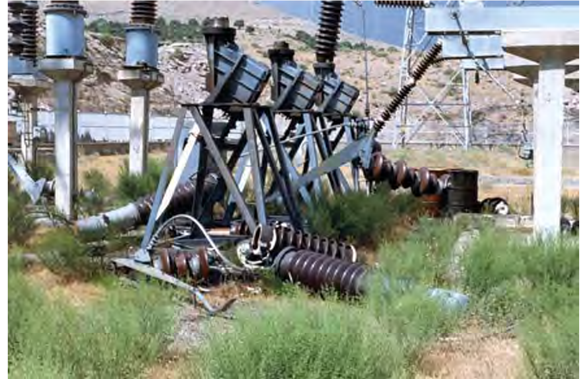
Overturned switchyard equipment with high center of mass caused by amplified ground shaking on fill, and ground movements (Sefid Rud dam, June 21, 1990, Manjil earthquake)
