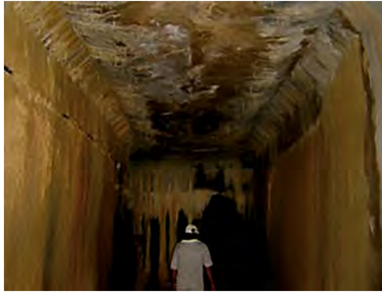
Leaching observed in the downstream face of a Dam and in the inner part of the dam gallery-(Andriolo's archive)
