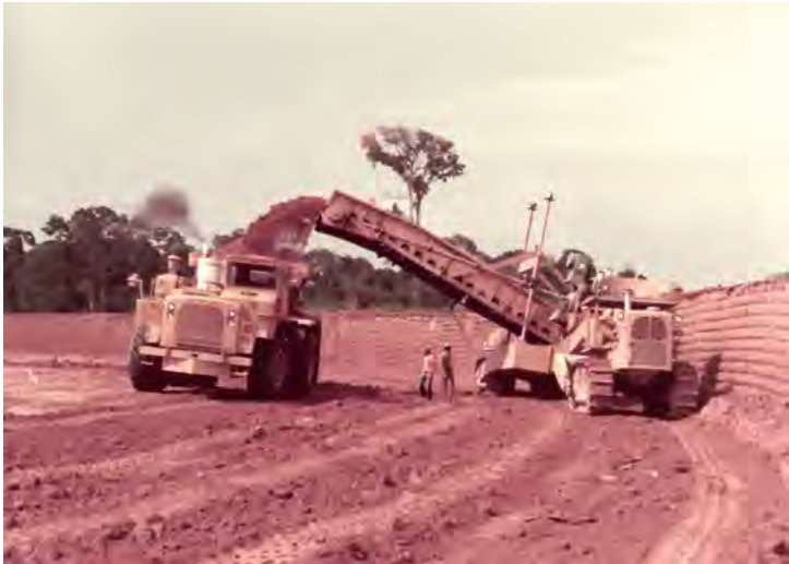
Earth excavation and handling more than 24.000.000 m 3 during the construction of Tucuruí Project – PA, Brazil (Courtesy from Ulysses Nunes Archive)
