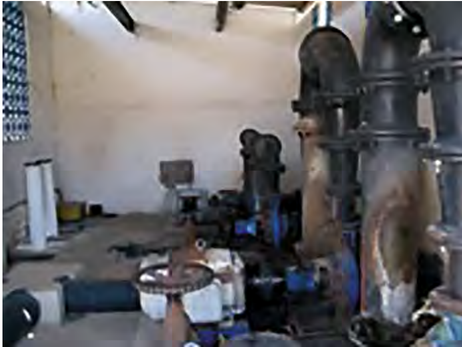
Poorly maintained mechanical and electrical equipment (Pictures from Andriolo's archives)
