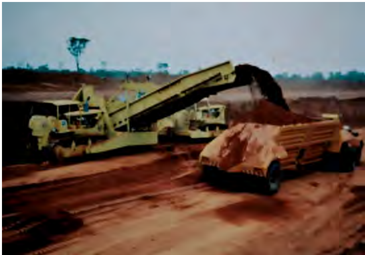
Earth excavation and handling more than 24.000.000 m 3 during the construction of Tucuruí Project – PA, Brazil (Courtesy from Ulysses Nunes Archive)
