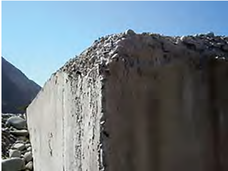
Freeze-thaw aspects on concrete showing some degradation of the elements (Andriolo's Archive)
