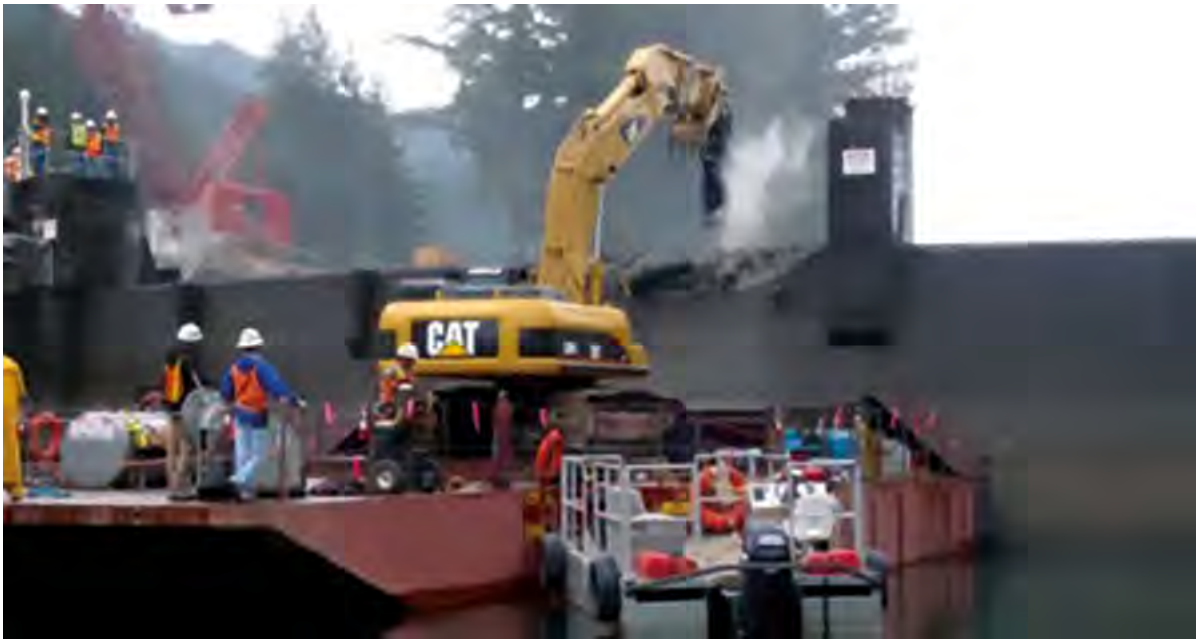
Hoe ram employed on a tracked vehicle floating on a barge immediately upstream from Glines Canyon Dam in Washington (photograph courtesy of Barnard Construction)
