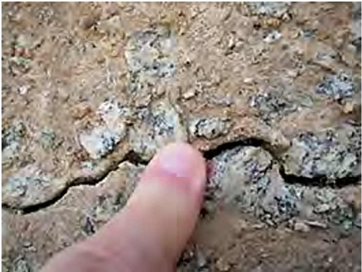
Concrete cracks due to chemical reactions (Pictures from Andriolo's archives)
