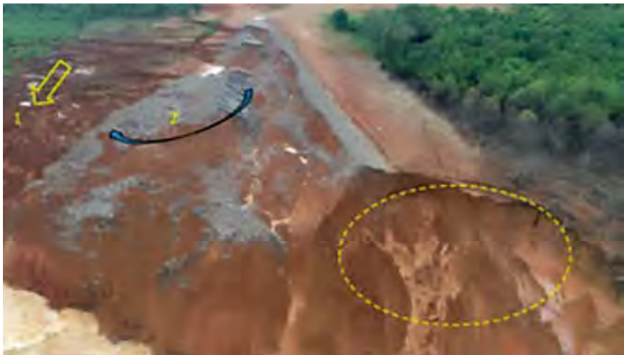
Beginning of water crossing the embankment (23 july 11:46)
