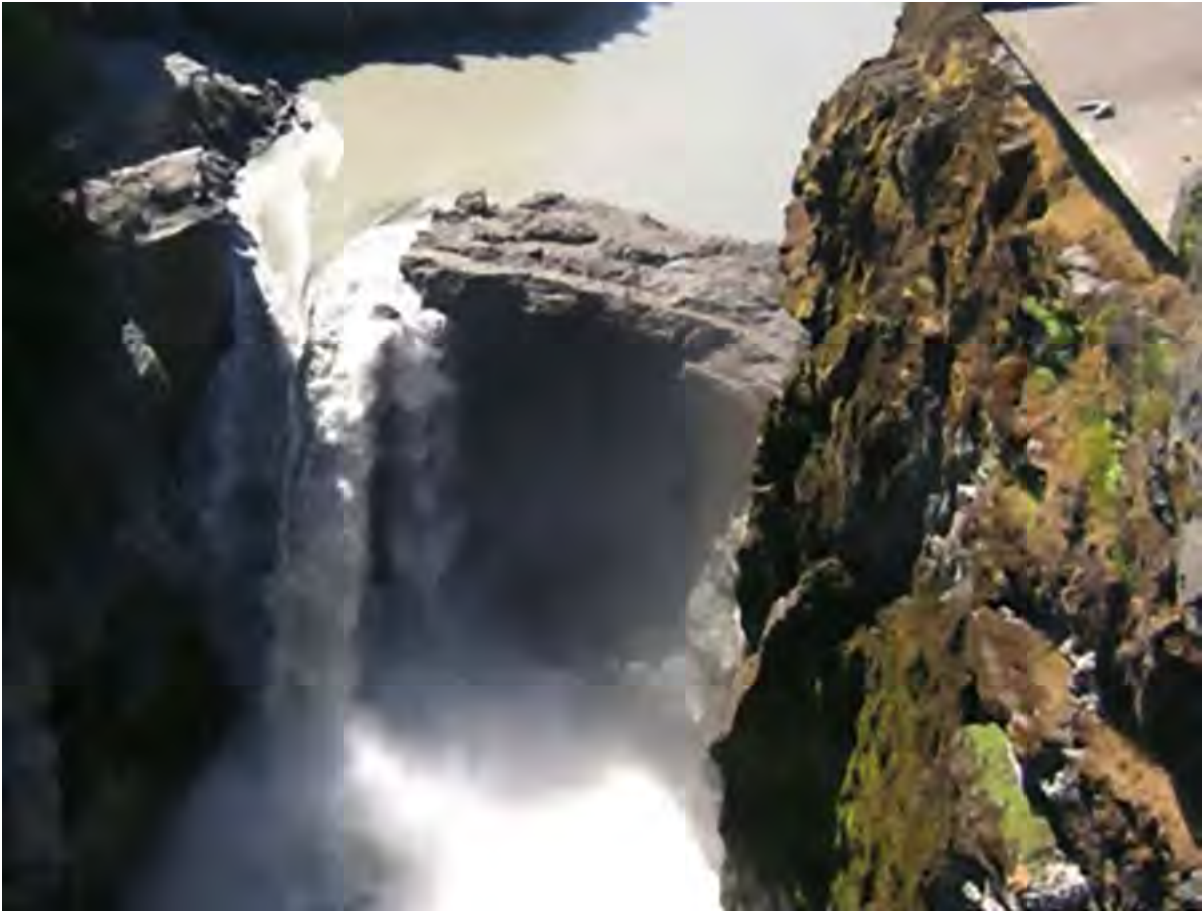
Demolition of the Glines Canyon arch dam section by blasting notches. A portion of the gated spillway is visible in the top-right corner of the photograph (photograph courtesy of Barnard Construction)
