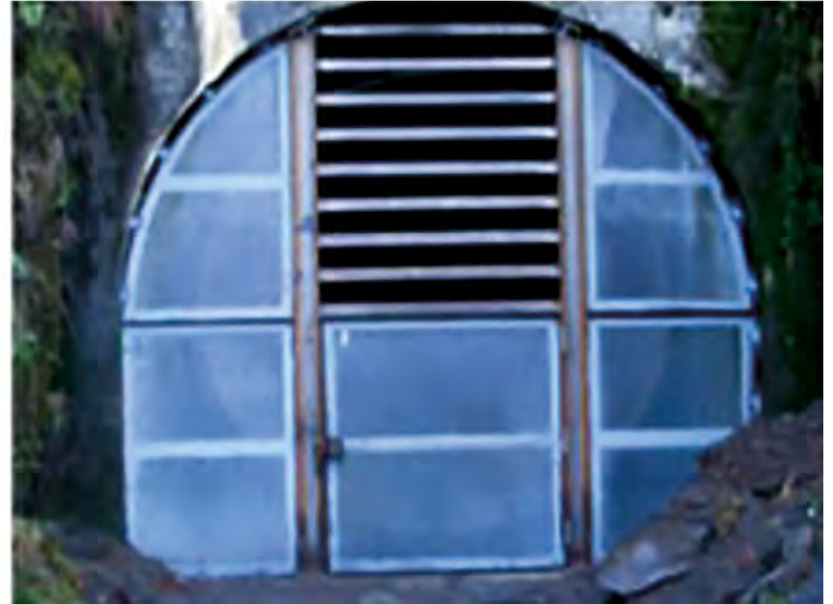
At Glines Canyon Dam, Washington, the upstream tunnel barrier (left) was blocked using precast concrete panels while the downstream tunnel barrier (right) was blocked using metal panels (photograph courtesy of Tom Hepler, Bureau of Reclamation.)
