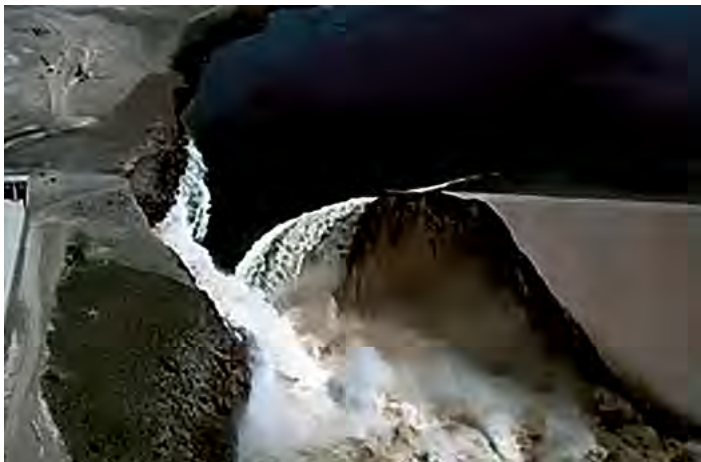
The sequence of the Teton Dam collapse (Courtesy from Bureau of Reclamation)
