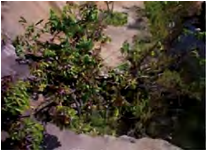
Trees and vegetation along the spillway that can create concentrated flow that can cause erosion (pictures from Andriolo's archives)
