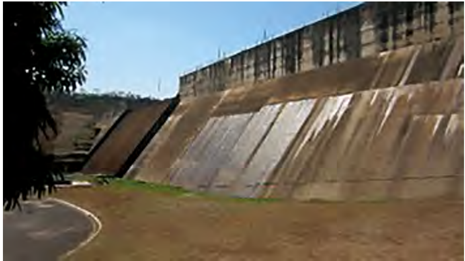
Poor quality of RCC in a dam due to inadequate construction joint surface treatment and/or inadequate water tightness system (Pictures from Andriolo’s archives)
