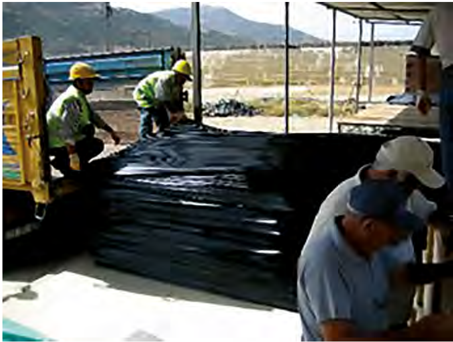
PVC Membrane used in a concrete precast panel for the Beydag RCC Dam in Turkey- (Andriolo's Archive)
