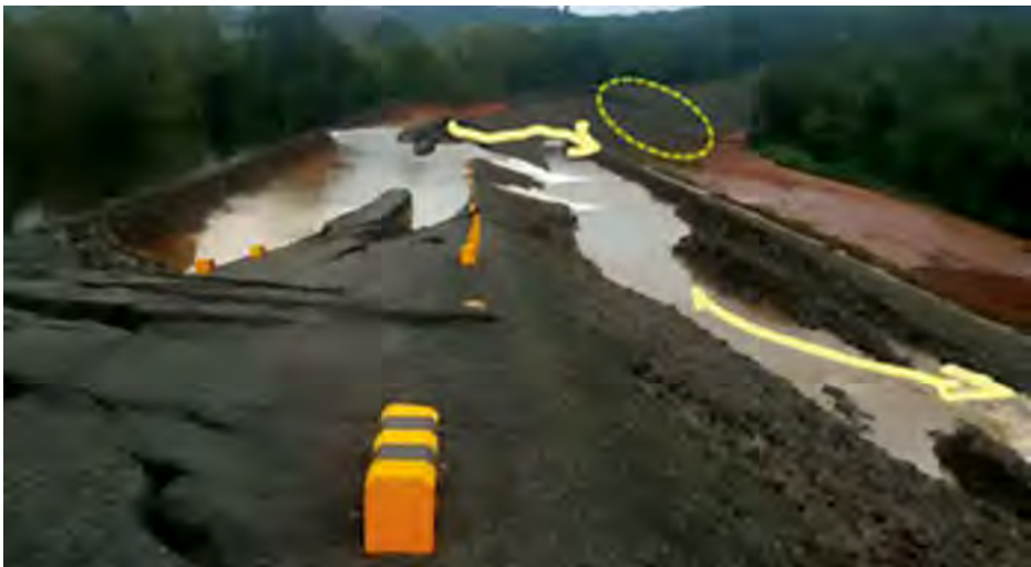
Initiation of the failure (23 july 04:30)
