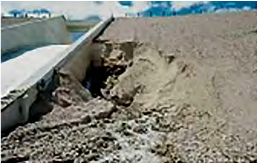
The third embankment slide on July 27, 1965
