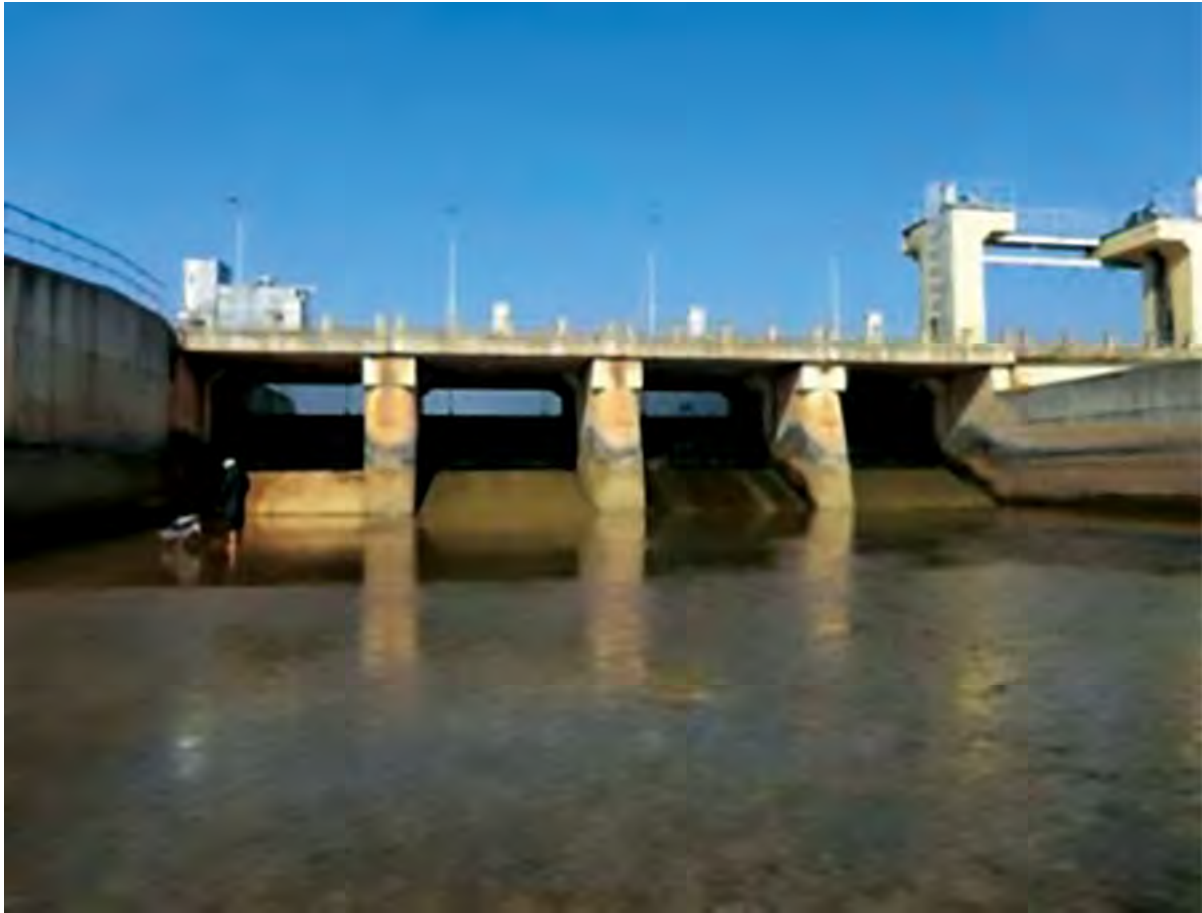
Gate leaves in apparently good conditions
