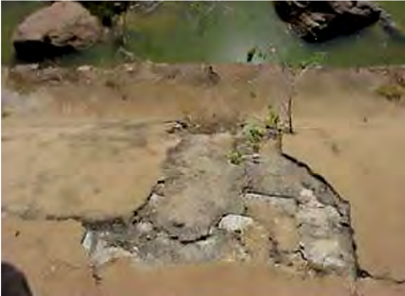
Concrete erosion on spillway surface due to poor concrete quality and lack of maintenance (Pictures from Andriolo's archives)
