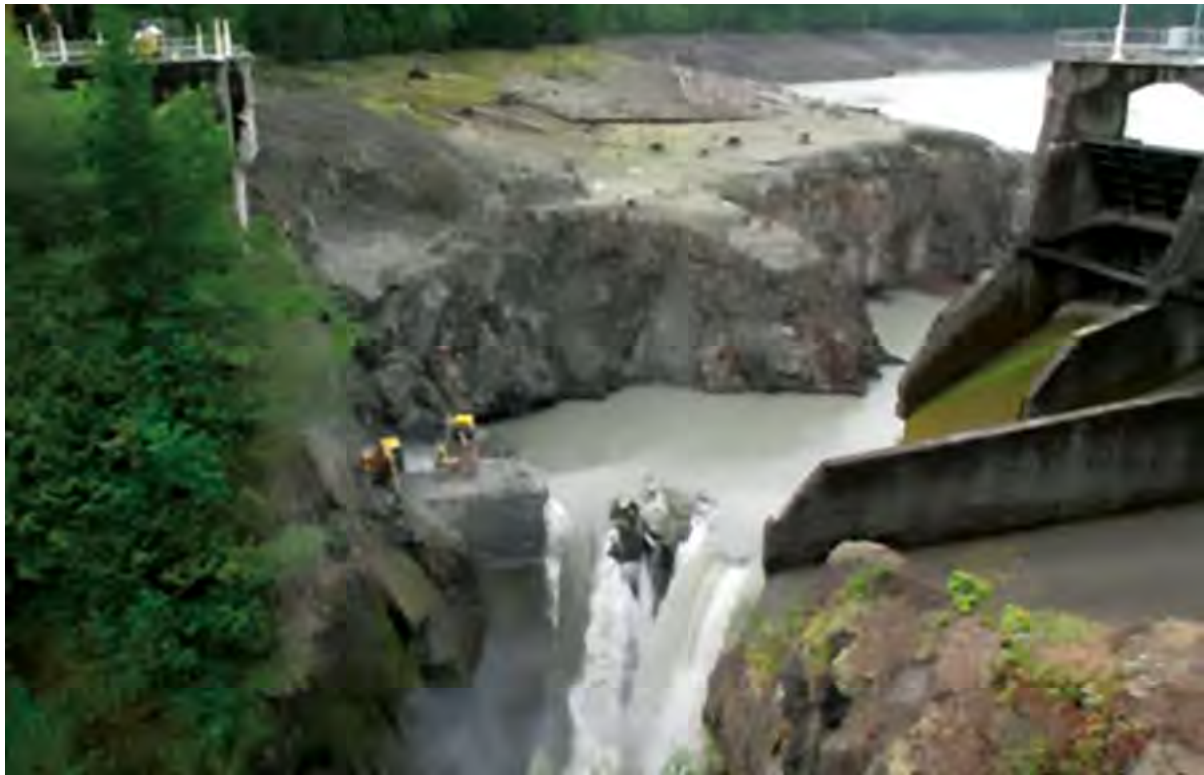
Drilling and blasting notches for excavation of the lower portion of Glines Canyon Dam in Washington (Photograph courtesy of National Park Service, July 1, 2012)
