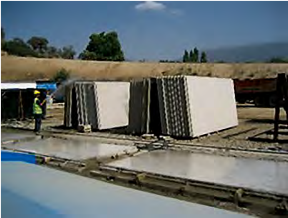
PVC Membrane used in a concrete precast panel for the Beydag RCC Dam in Turkey- (Andriolo's Archive)
