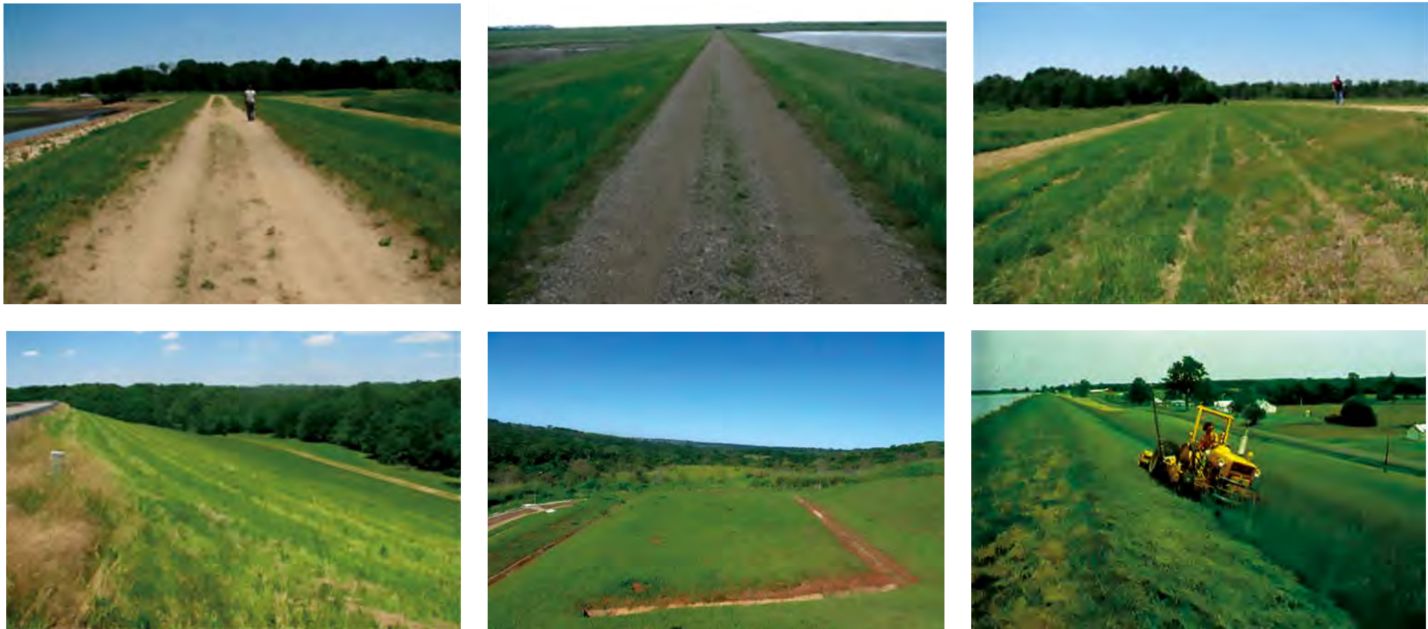
Figures showing an Acceptable Vegetation Control (From Refs. [09-04] to [09-08])
