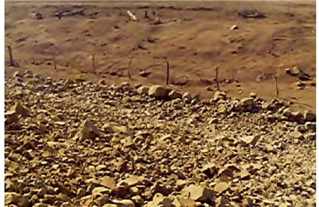
Riprap erosion protection (upstream and downstream zones) on an embankment slope (Pictures from Andriolo's archives)
