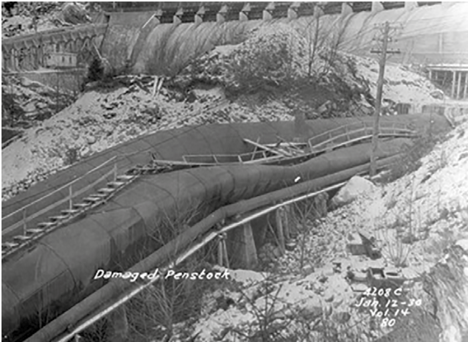
Buntzen Hydro Dam - Damaged Penstock - City of Vancouver Archives
