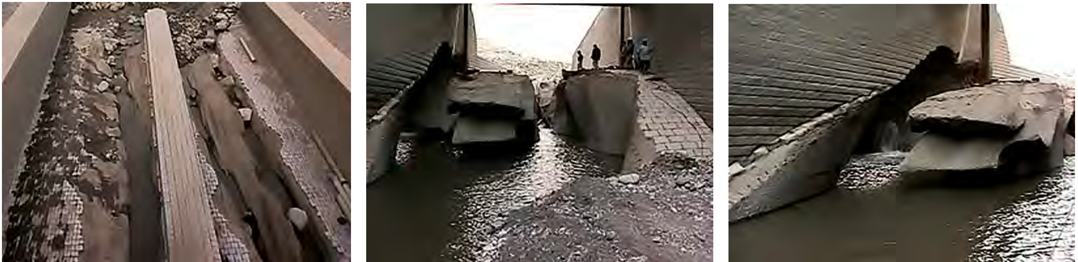
Figures showing huge erosion in a concrete spillway structure (Pictures from Andriolo's archives)
