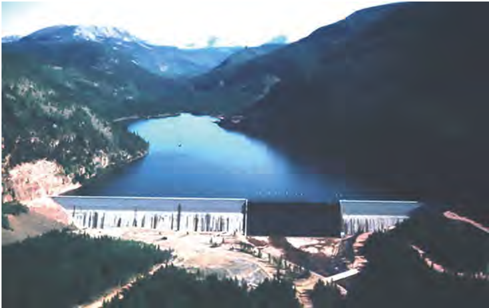
Aerial view of the completed Upper Stillwater Dam, showing the downstream face and seepage from cracks following the first winter and first filling
