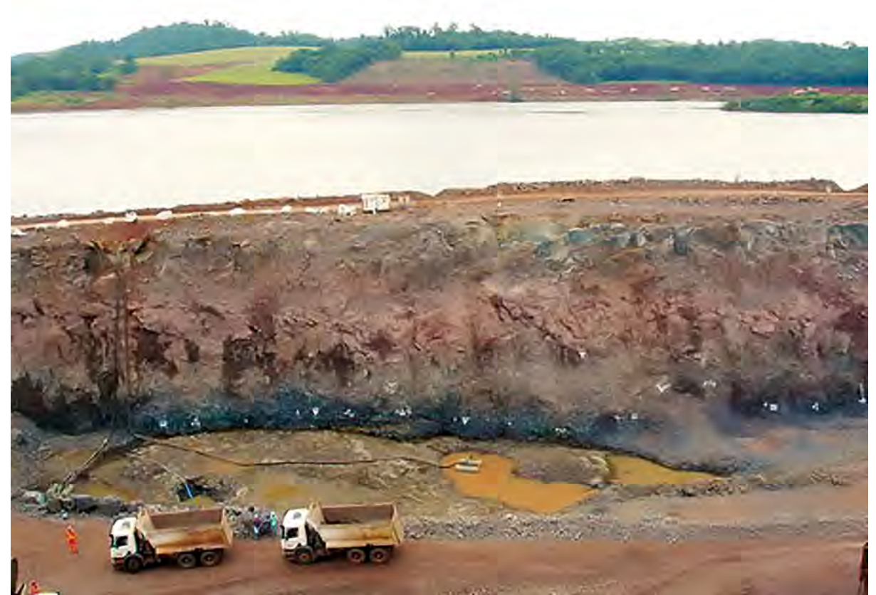
This picture shows the same situation of contact between basaltic flows showing the formation of an important low strength joint whose persistence is much greater than the dam itself
