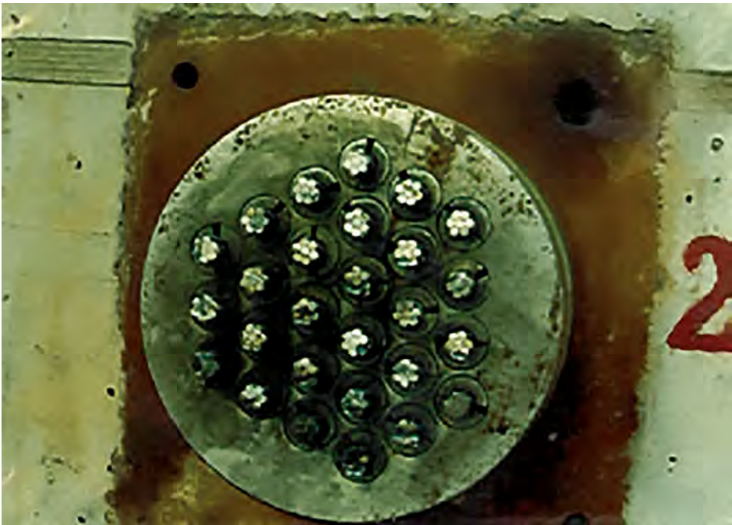
Ducts and tendons for post-tensioning a pier – Itaipu Spillway Piers, 1979 (Andriolo's Archive) [03-01]
