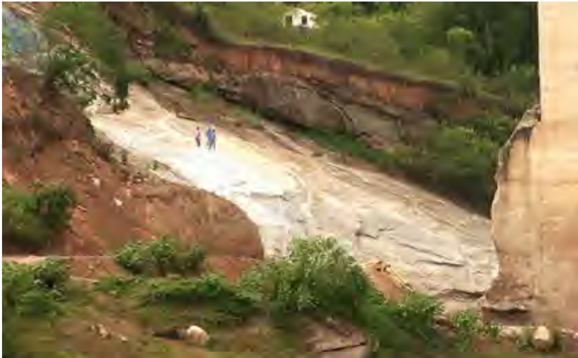
Relief joint in Camará Dam
