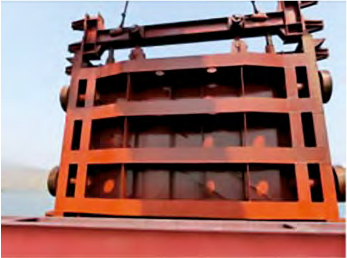
The stoplog gate leaf was in sound condition
