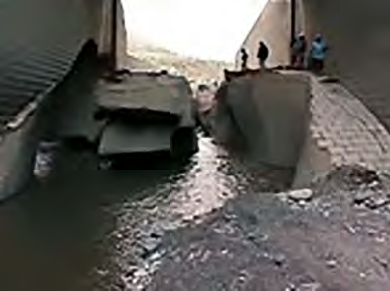
Damages in the structures and gates of Chavimochic Dam Spillway (Pictures from Andriolo's Archive)
