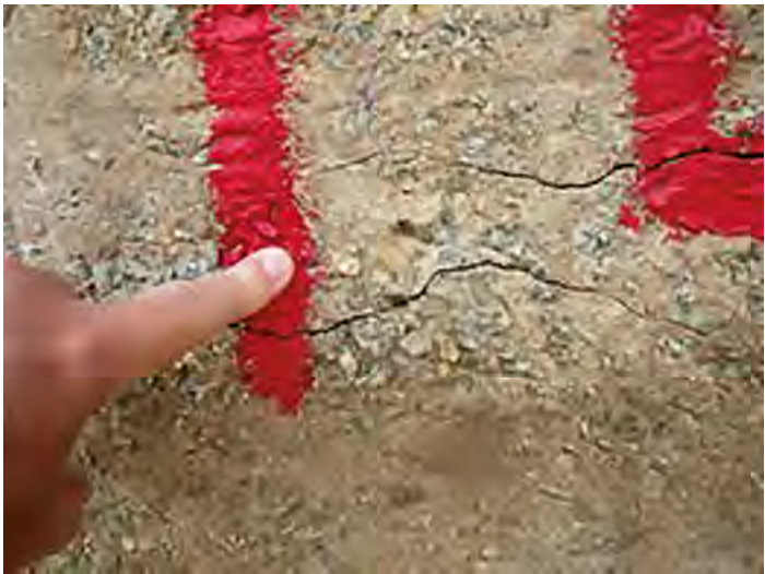
Concrete cracks due to chemical reactions (Pictures from Andriolo's archives)
