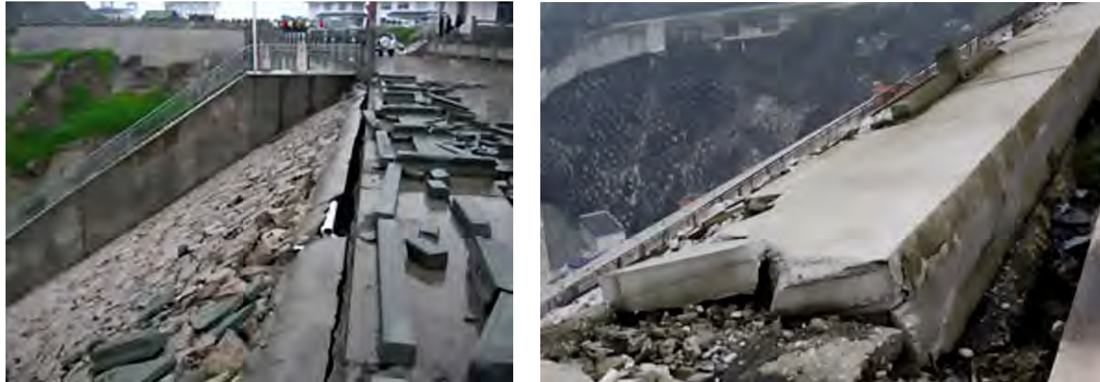
Damages observed on Zipingpu CFR Dam [01-17 & 01-18]
