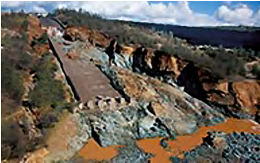
The large flow and the damage in the Oroville Spillway
