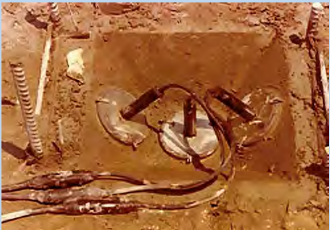
Sequence of installation of a stress meter set in the mass concrete at Itaipu Project (From Andriolo's Archive, 1978)
