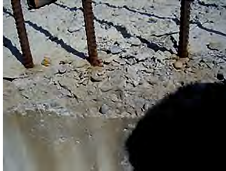
Freeze-thaw aspects on concrete showing some degradation of the elements (Andriolo's Archive)
