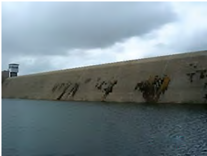
Poor quality of RCC in a dam due to inadequate construction joint surface treatment and/or inadequate water tightness system (Pictures from Andriolo’s archives)
