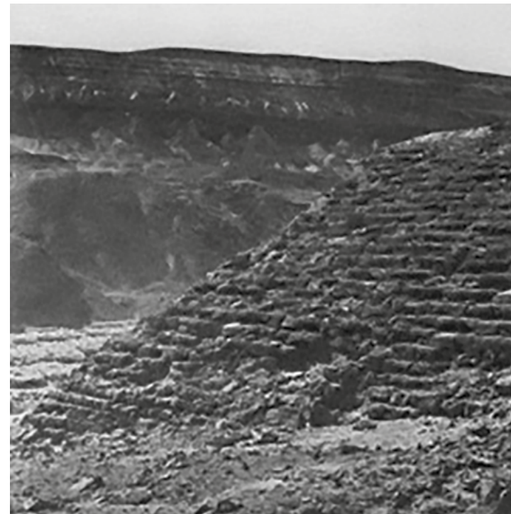
Upstream face of northern wall, photo of 1982. Remains of the poorly designed Sadd el-Kafara [01-03]
