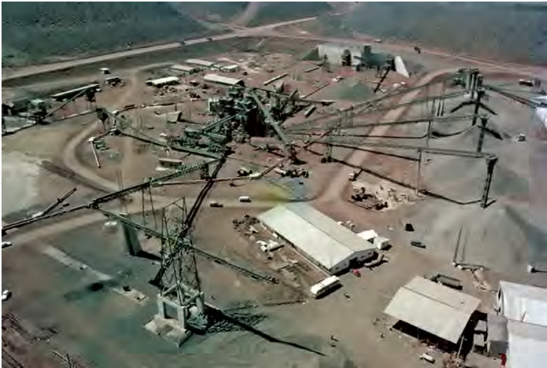
View of the aggregate processing installations on the left bank of Parana River in September 1977, before beginning the concrete works of the diversion structures
