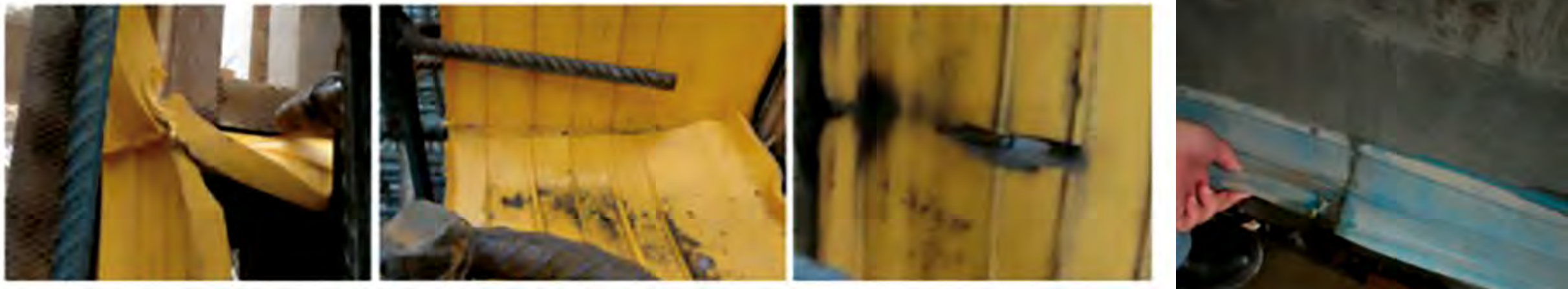
Mistakes that need to be avoided during the use of PVC waterstops [03-03]
