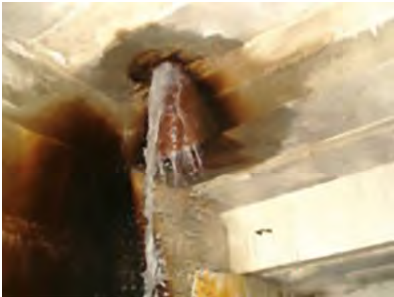
Poor quality of RCC in a dam due to inadequate water tightness system (Pictures from Andriolo's archives)
