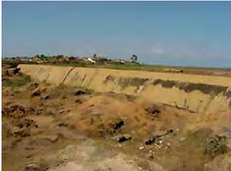
Concrete erosion on spillway surface due to poor concrete quality and lack of maintenance (Pictures from Andriolo's archives)
