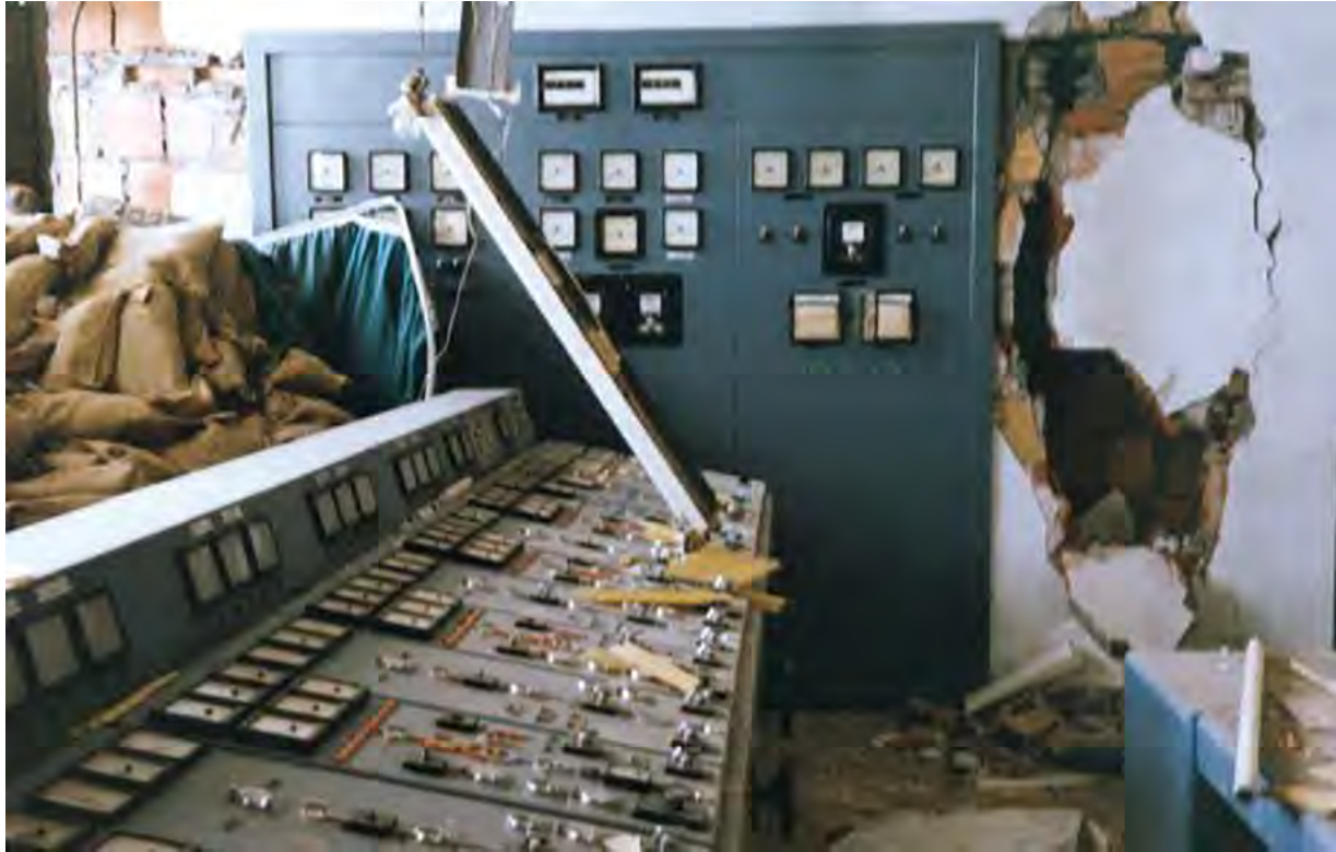
Non-structural elements falling on panel in control room of powerhouse of Sefidrud dam project and electrical cabinet attached to infill wall (June 21, 1990, Manjil earthquake)
