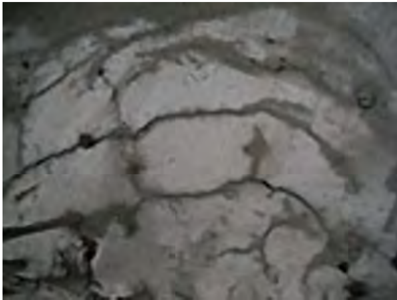
Concrete plastic settlement cracks due to poor vibration during the pouring (Pictures from Andriolo's archives)
