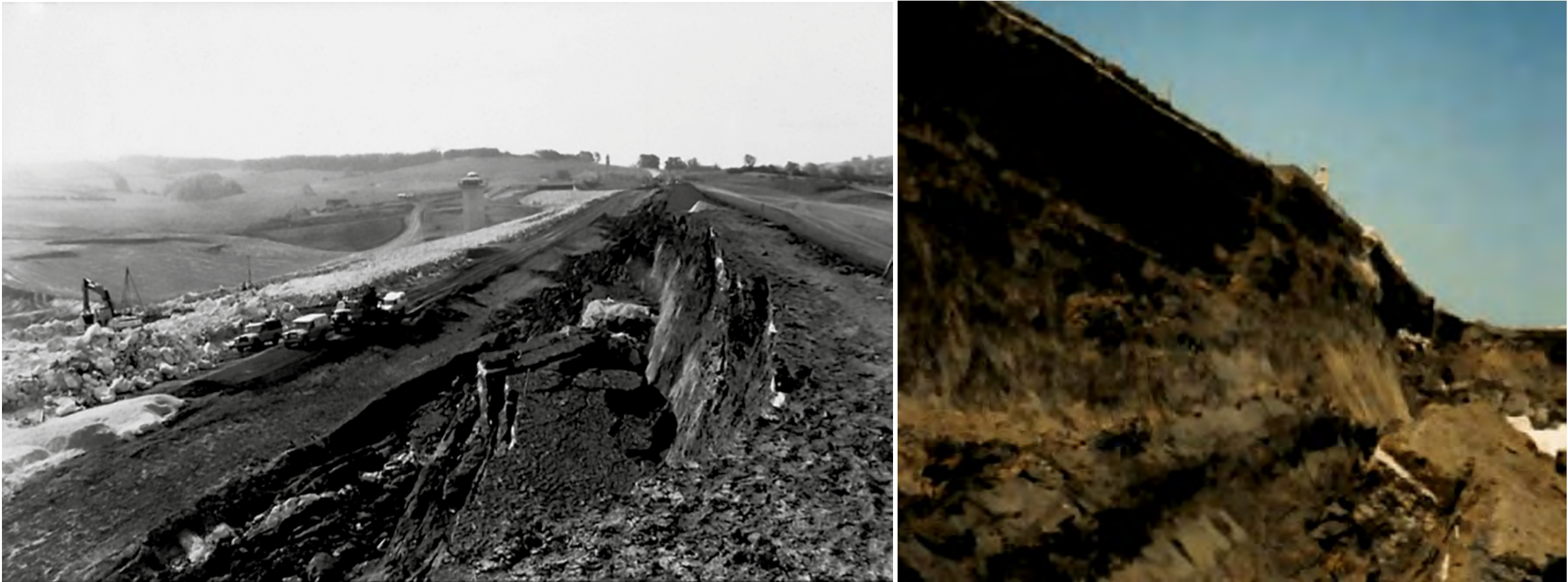
Partial collapse of Carsington Dam in 1984
