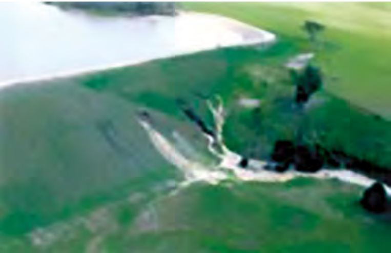
Embankment dams in initial pipping (from Refs. [09-06 to 09-08])
