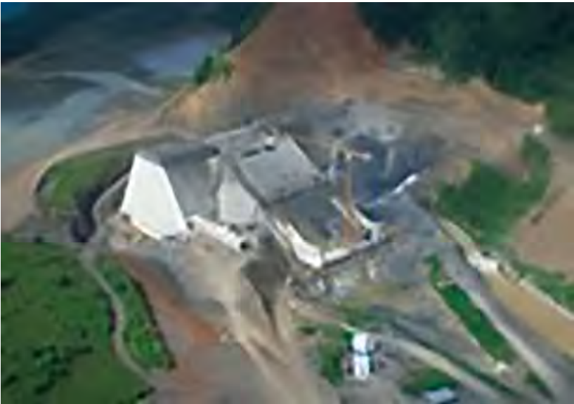
The repairs at El Guapo Dam with a new Spillway (Pictures from the reference above)
