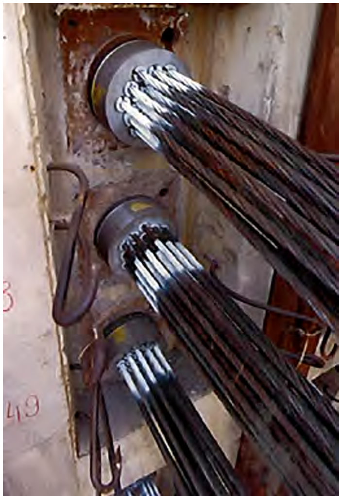
Ducts and tendons for post-tensioning a pier – Itaipu Spillway Piers, 1979 (Andriolo's Archive) [03-01]
