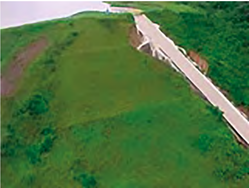
Damages in the El Guapo Dam around the Spillway (Pictures from the reference above)
