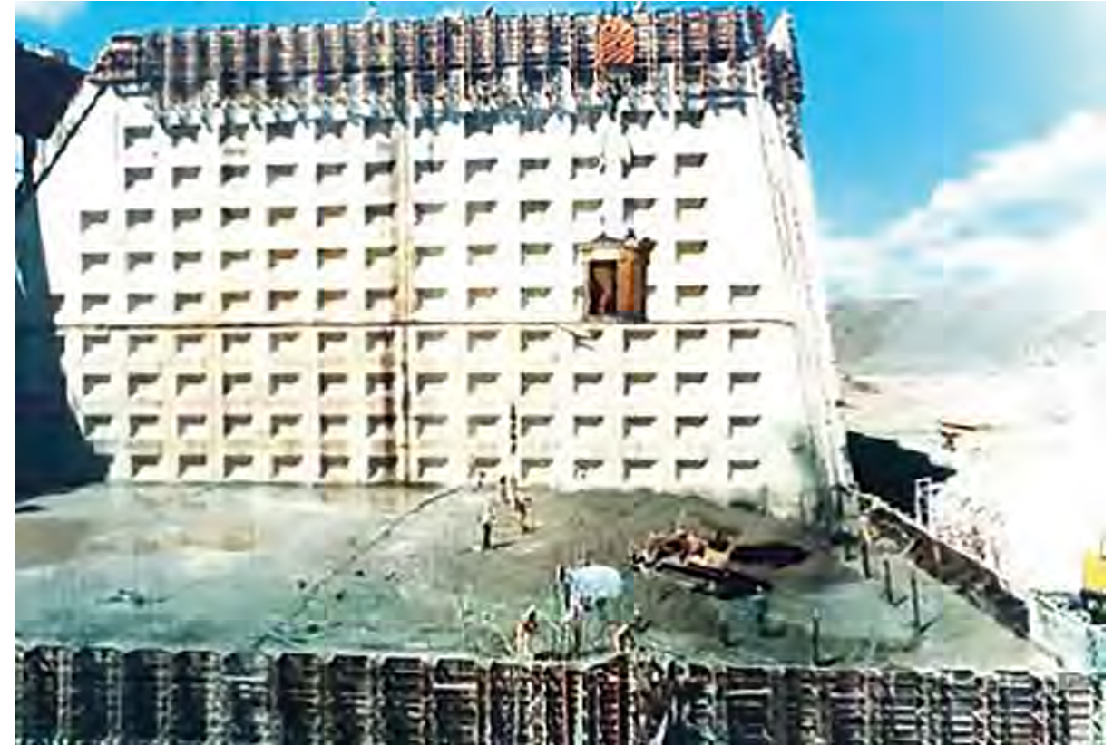
Shear keys in the concrete Tucurui Dam – Brazil – (Andriolo's Archive)
