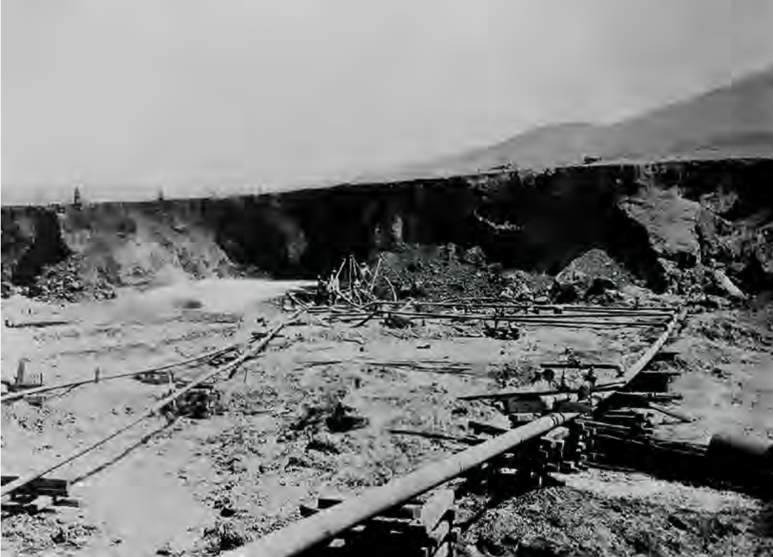
The original San Fernando Reservoir was constructed by the City of Los Angeles between 1911-17 using hydraulic “puddled fill technique”
