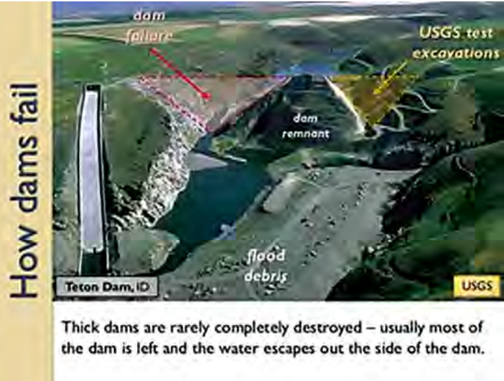
The sequence of the Teton Dam collapse (Courtesy from Bureau of Reclamation)
