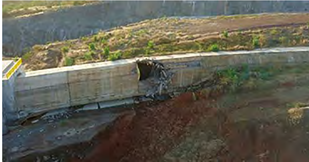
Concrete conduit failure, and concrete aspect after the damage - From the References
