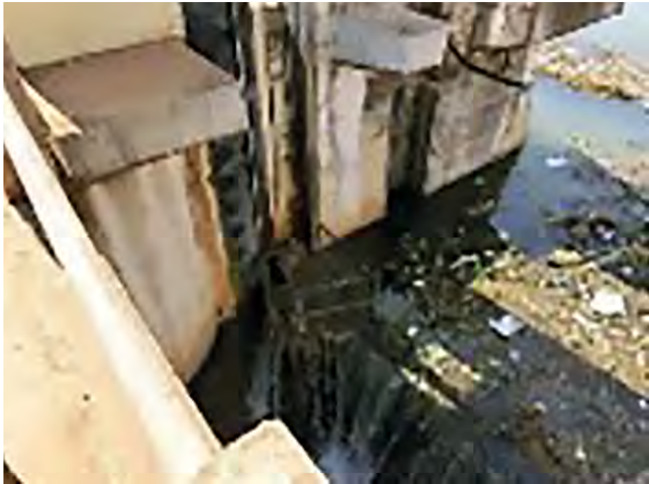
Failure of radial gate of run-of-river power plant due to rock falling on arm whose support has not been designed for transverse loads (May 12, 2008, Wenchuan earthquake)
