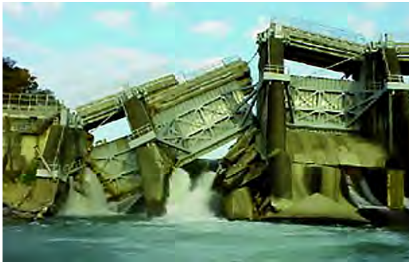
The Shi-Kang Dam built in 1977 and failed in 1999, due to the action of the Chi-Chi Earthquake
