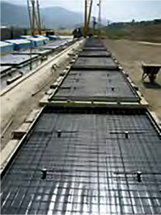
PVC Membrane used in a concrete precast panel for the Beydag RCC Dam in Turkey- (Andriolo's Archive)
