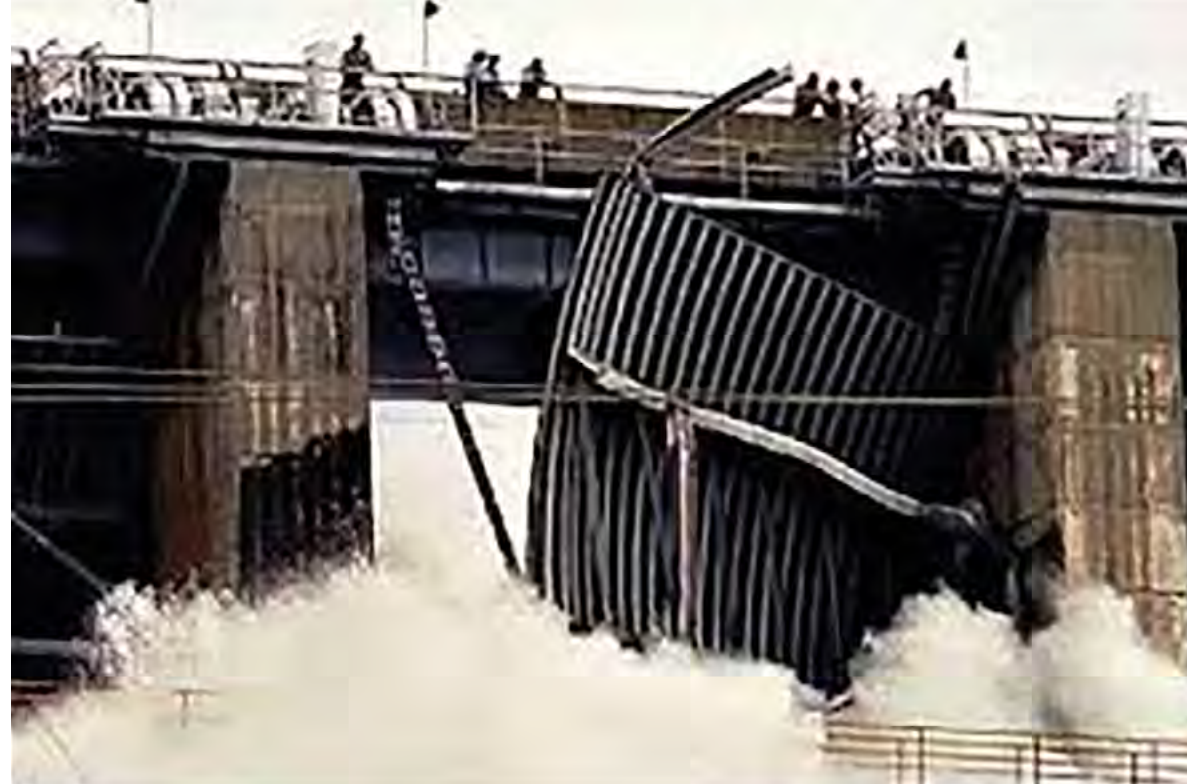
Radial gate at Folsom dam during and after the failure
