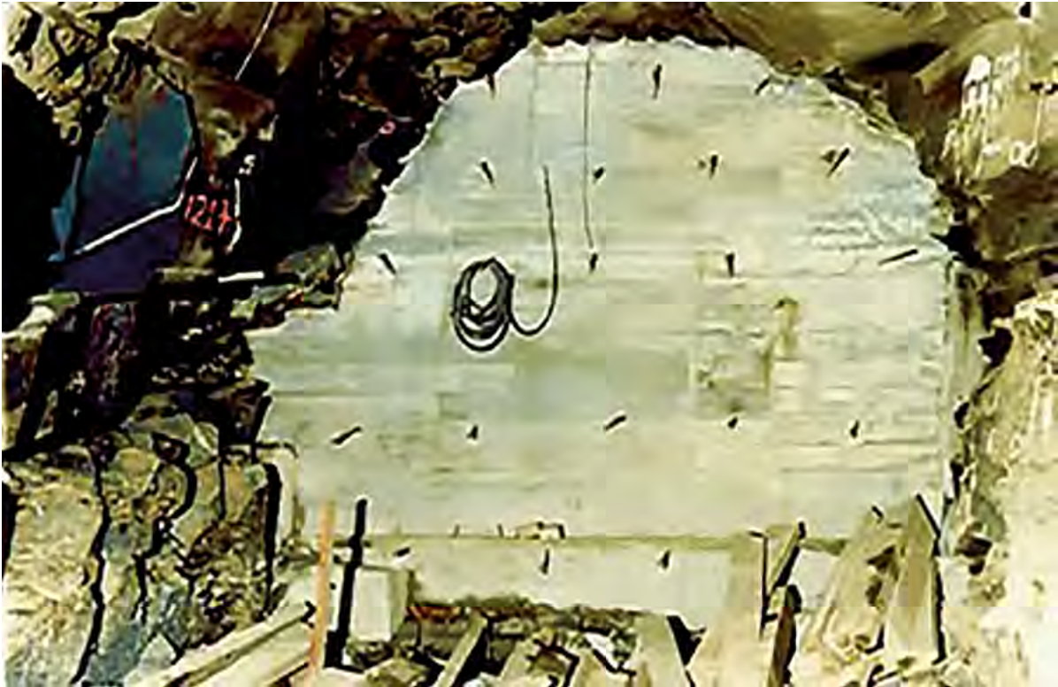
The picture shows one of the shear key tunnels partially concreted. The discontinuity is at half height of the tunnel
