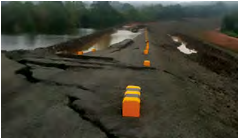
Beginning of water crossing the embankment (23 july 11:46)
