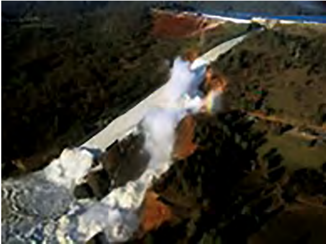
The large flow and the damage in the Oroville Spillway
