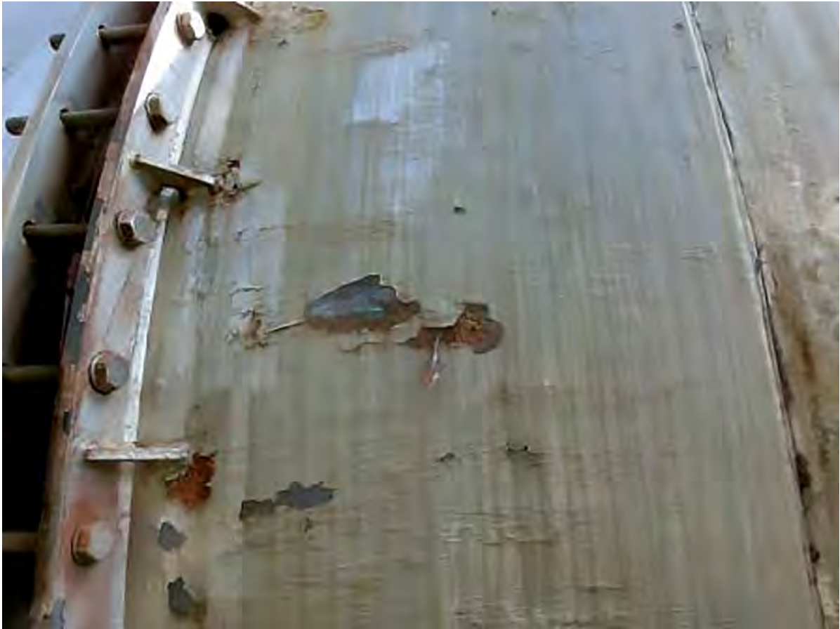
The trace of water leak can cause damages to the protection paint (from Ref. [09-02])
