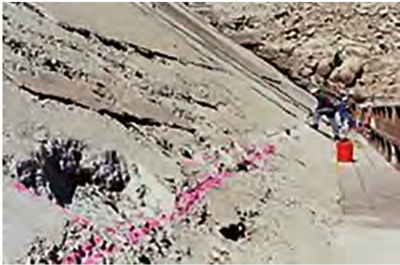
Views of the damages of the concrete face on Salt Springs Dam and the repair using a PVC Membrane
