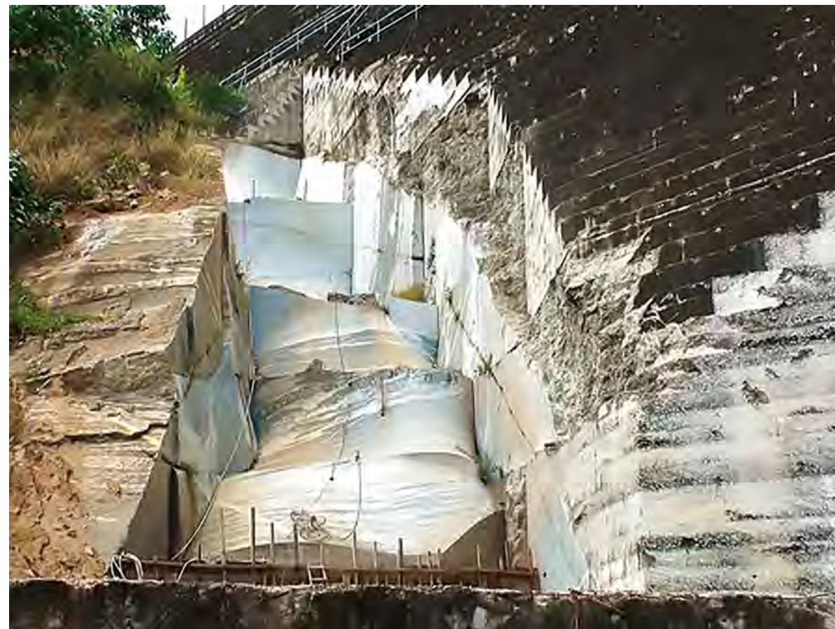
Cable sawing in the concrete and in the rock in the left abutment
