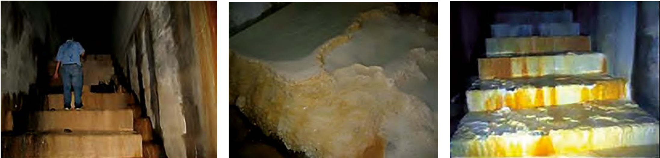
Leaching observed in the downstream face of a Dam and in the inner part of the dam gallery (Andriolo’s archive)
