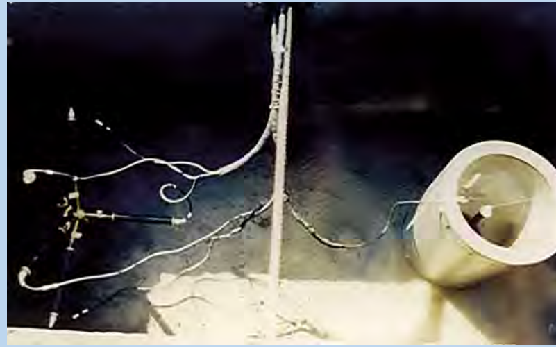
Installation of a strain meter spider and autogenous box in a confined zone at Tucuruí Project (From Andriolo's Archive, 1982)
