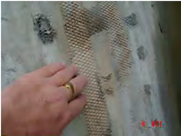
Expanded metal meshes used as form (Andriolo's archive).
