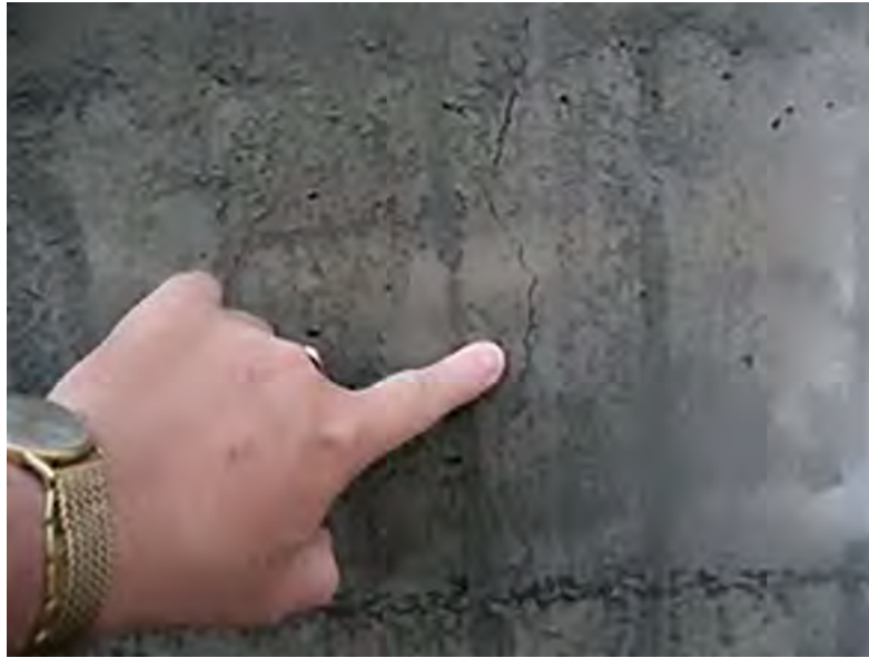
Thermal cracks observed in different concrete structures (Andriolo's Archive)
