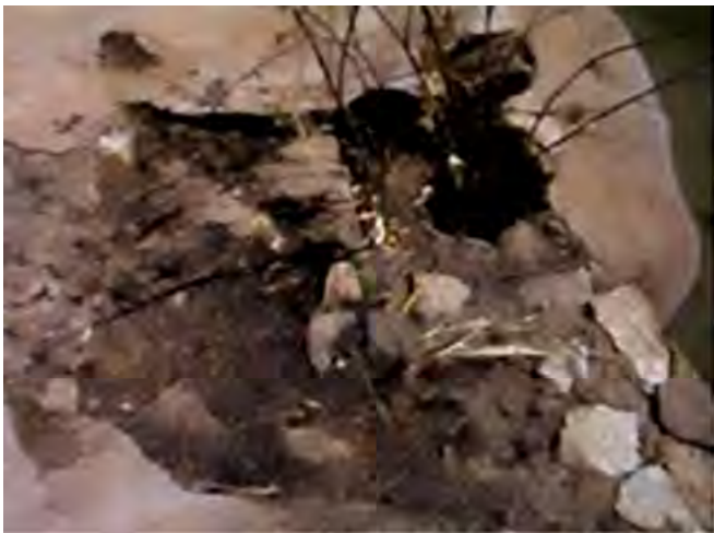
Trees and vegetation along the spillway that can create concentrated flow that can cause erosion (pictures from Andriolo's archives)
