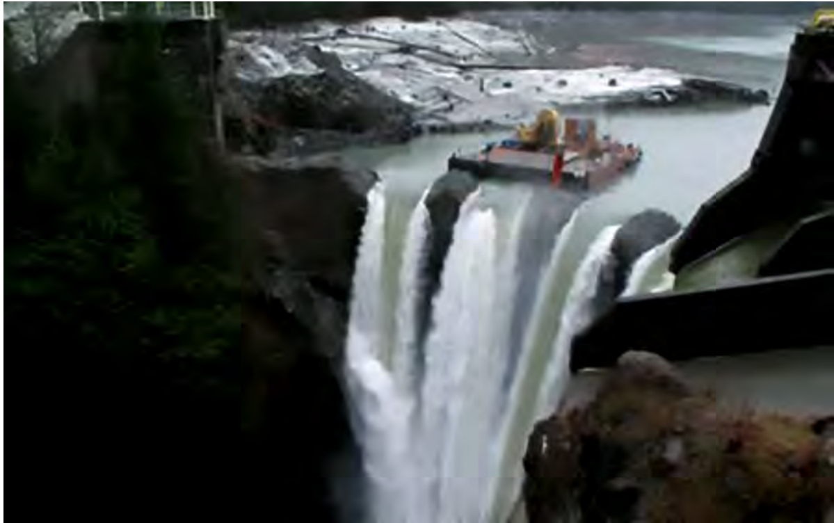
Mechanical excavation of the upper portion of Glines Canyon Dam in Washington, using a hydraulic excavator on a barge. (Photograph courtesy of National Park Service, January 14, 2012)
