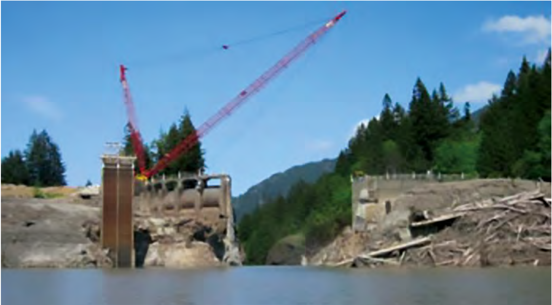
A large ring crane was employed at Glines Canyon Dam, WA (photograph courtesy of Tim Randle, Bureau of Reclamation)
