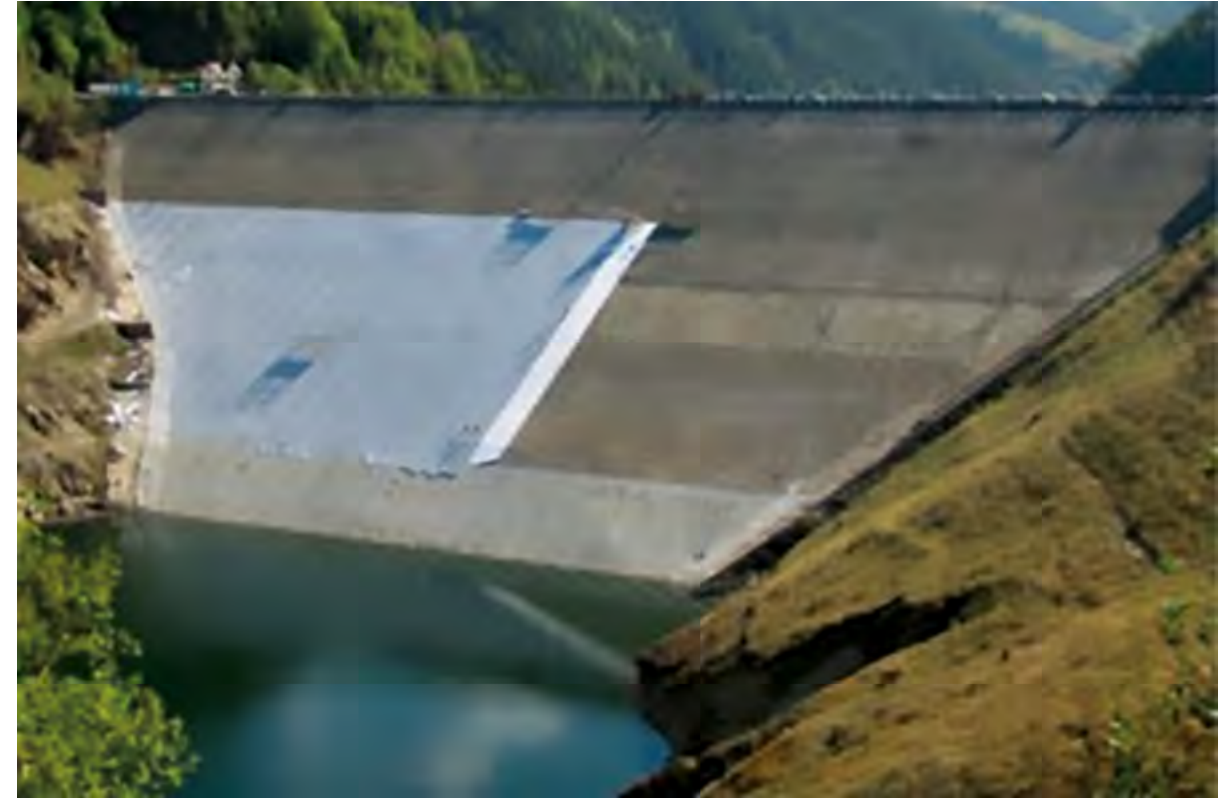
PVC geocomposite sheets under installation on anti-puncture geotextile (the white material) in stage 2 at Pecineagu CFRD in Romania - 2012 [03-29]
