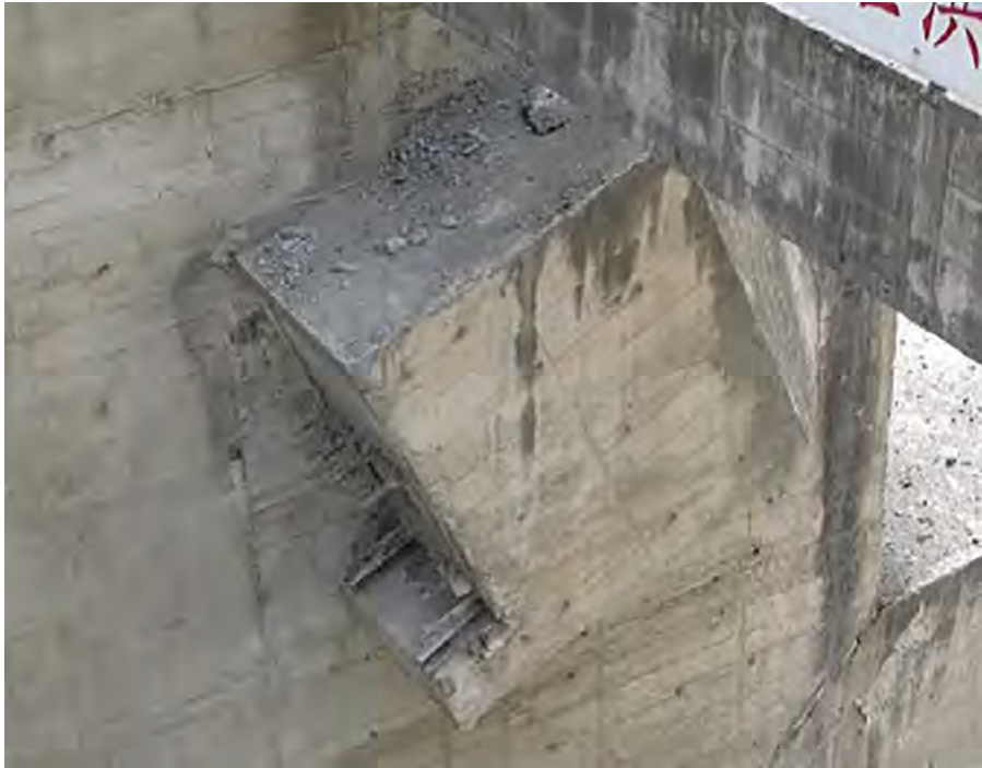
Failure of radial gate of run-of-river power plant due to rock falling on arm whose support has not been designed for transverse loads (May 12, 2008, Wenchuan earthquake)
