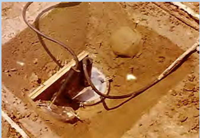
Sequence of installation of a stress meter set in the mass concrete at Itaipu Project (From Andriolo's Archive, 1978)
