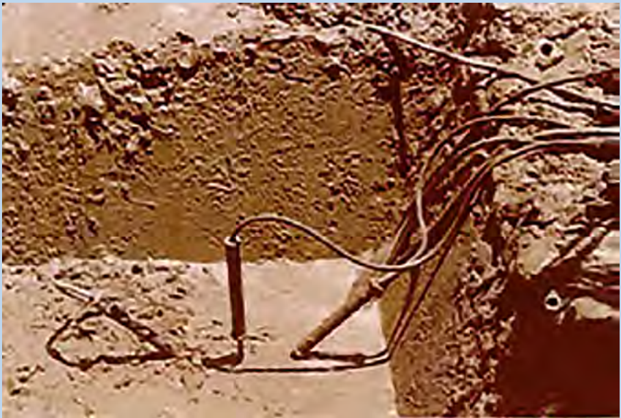
Sequence of installation of a strain meter spider and autogenous box in the mass concrete at Itaipu Project (From Andriolo's Archive, 1978)
