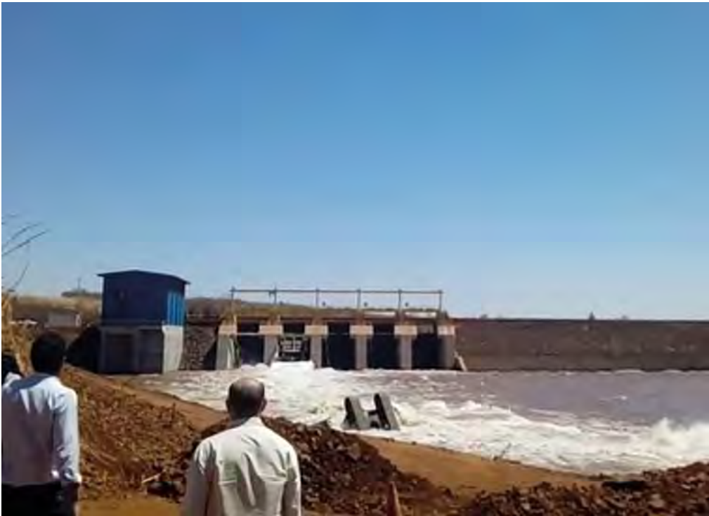
Moment of the Rupture of the Ype Dam Spillway
