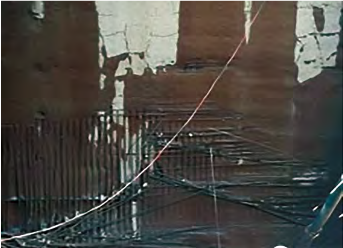
Inadequate covering of the rebars, in a Spillway wall, that was noted after a first water flow (Andriolo’s Archive)
