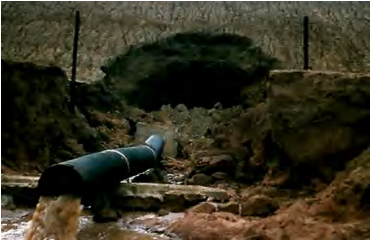
Embankment dams in initial pipping (from Refs. [09-06 to 09-08])
