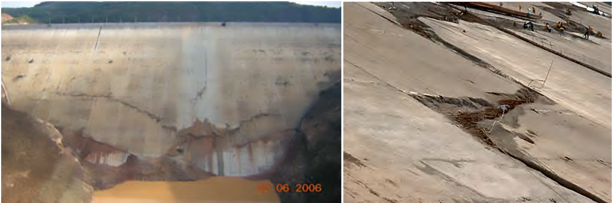
The damages at Campos Novos CFRD
