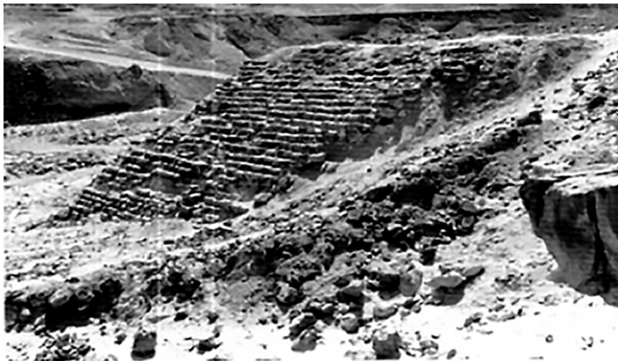
Upstream face of northern wall, photo of 1982. Remains of the poorly designed Sadd el-Kafara [01-03]
