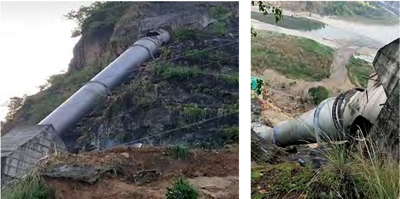
Penstock of the power house that was burst during the trial step
