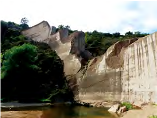
Views of the Malpasset Dam after construction, as operating, and after the collapse
