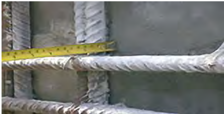
Poor installation of the rebars. This need be avoided. (courtesy by Pedro Augusto Cassimiro de Araujo)
