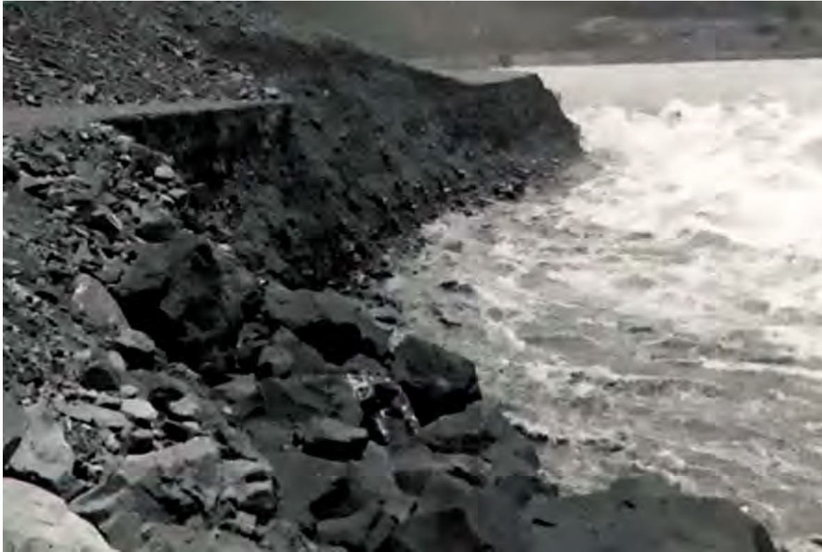
Riprap erosion protection (upstream and downstream zones) on an embankment slope (Pictures from Andriolo's archives)
