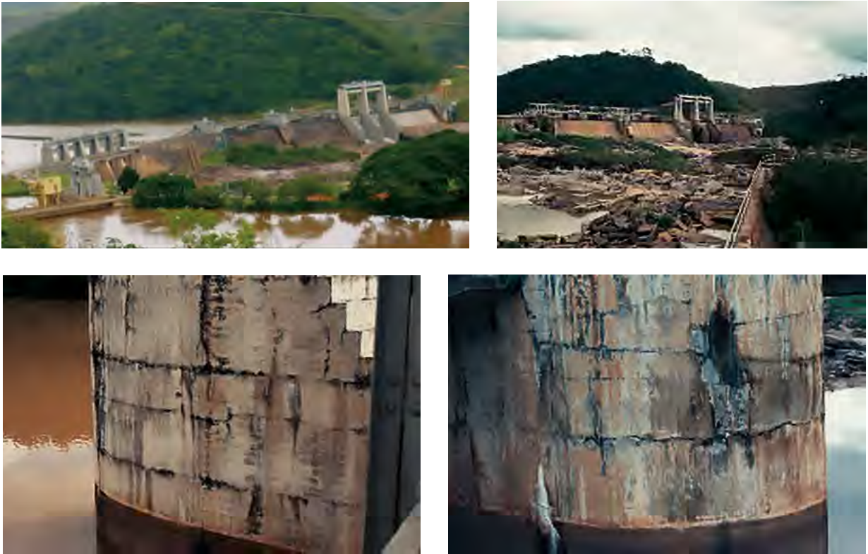
Ilha dos Pombos Dam that had been finished by 1924, (Brazil) and had shown RAA expansions (Andriolo’s Archive)
