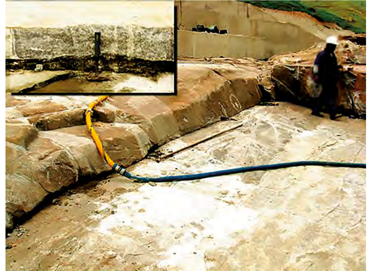
Another feature that also draws attention are the relief joints, very common mainly in granites, gneisses, migmatites, and which follow the topographic shape and when close to the riverbed become sub horizontal
