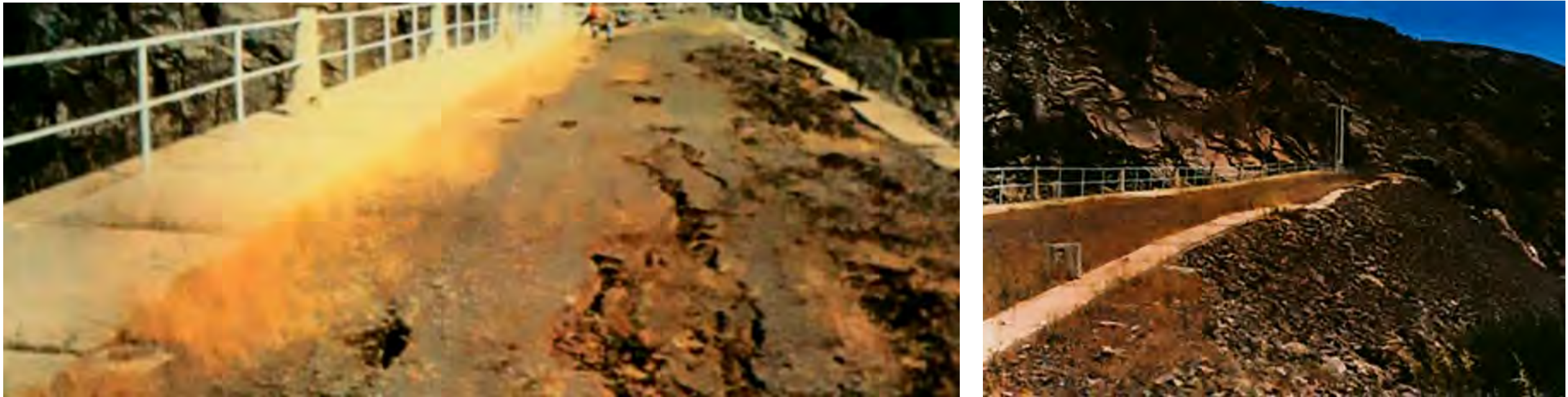
Cogoti CFRD in Chile before (top) and after the 14 October 1977 Punitaqui earthquake (middle); cracks on dam crest (bottom) (Photographs courtesy G. Noguera, Chile)
