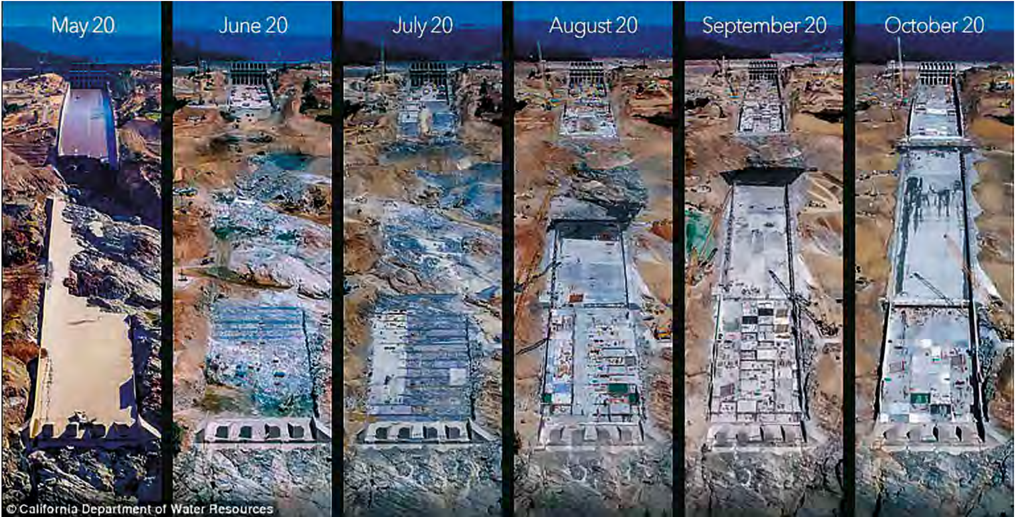
Oroville Spillway repair development since the damage (Courtesy from California Department of Water Resources)
