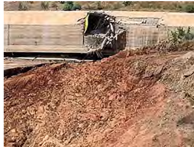
Concrete conduit failure, and concrete aspect after the damage - From the References
