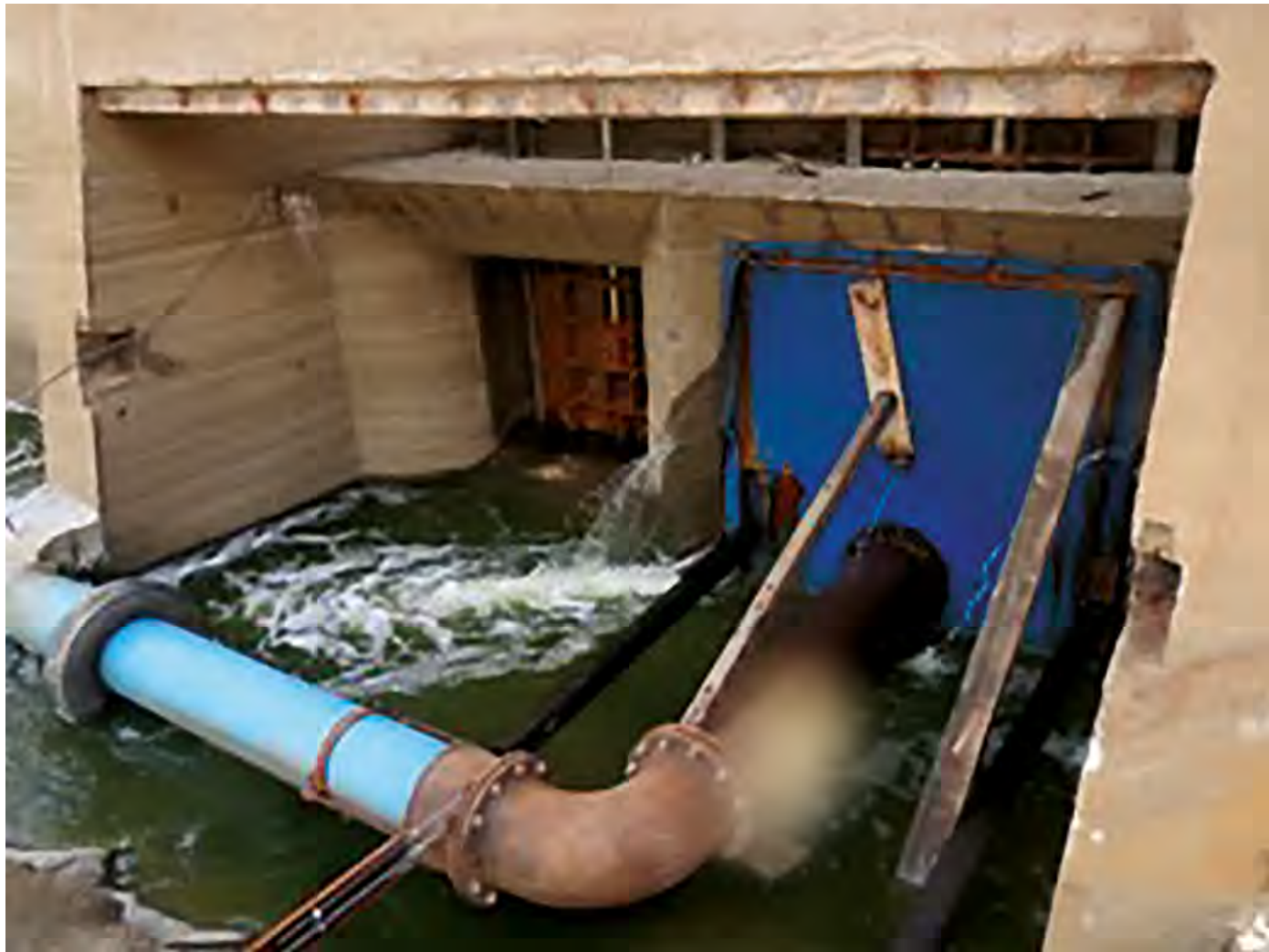
Inadequate support for pipes (Pictures from Andriolo’s archives)
