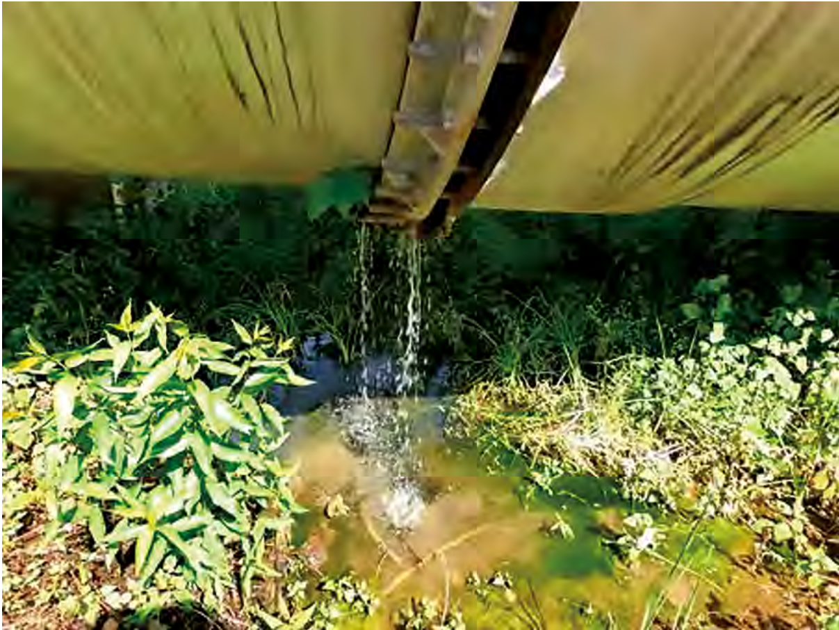
Water leaks from some expansion joints (from Ref. [09-02])
