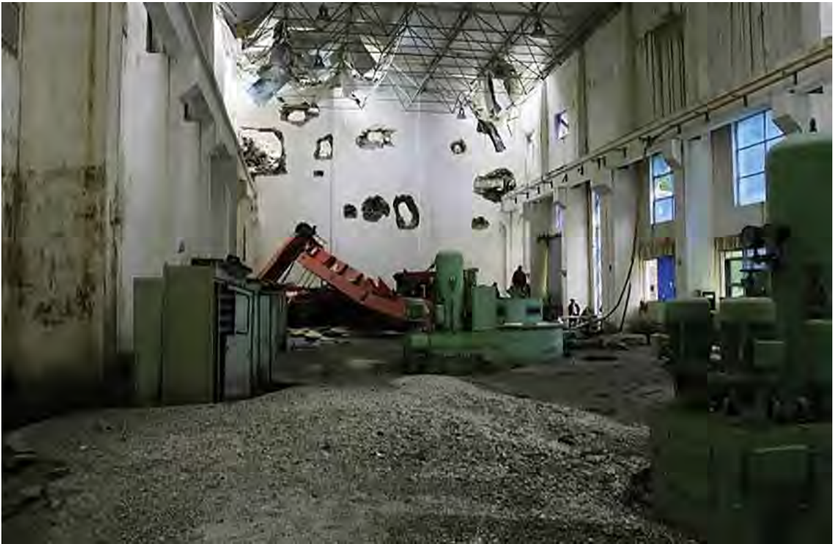
Damaged crane, end wall and roof of powerhouse of Shapai arch-gravity dam project caused by rockfall; sediments were deposited due to penstock failure and powerhouse earthquake, China)
