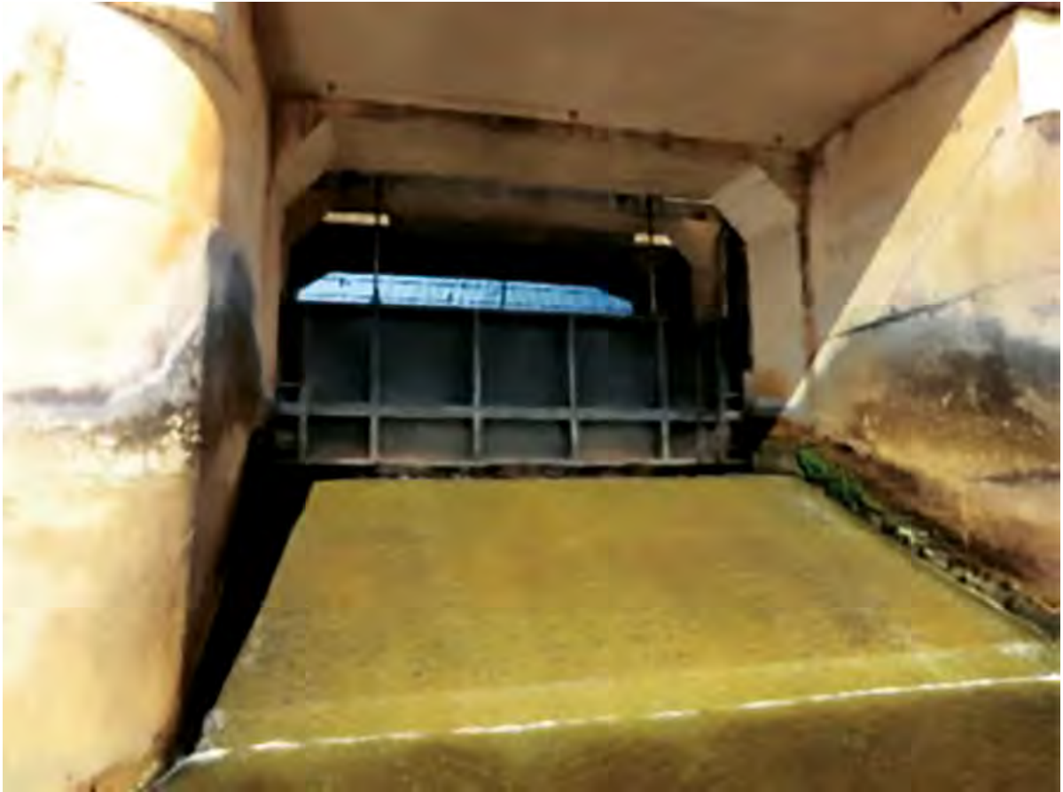
Gates presenting water leak
