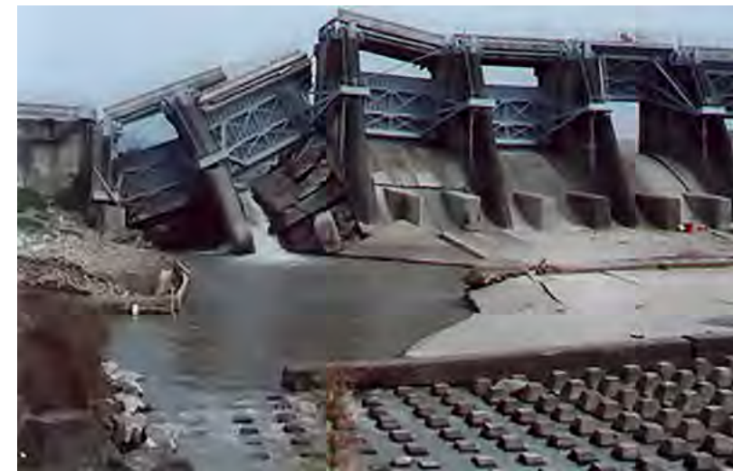
The Shi-Kang Dam built in 1977 and failed in 1999, due to the action of the Chi-Chi Earthquake
