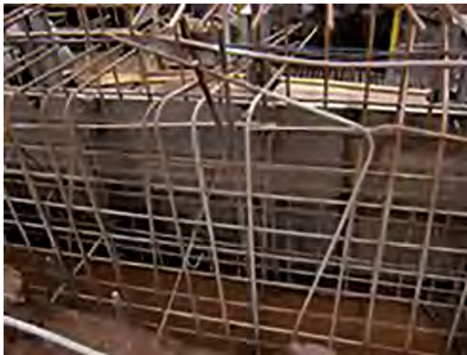
Poor installation of the rebars. This need be avoided. (courtesy by Pedro Augusto Cassimiro de Araujo)
