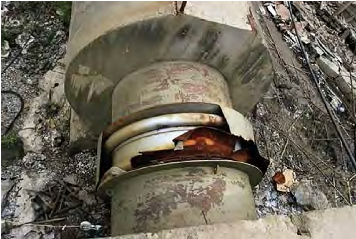
Failure of penstock near Shapai powerhouse: detail of damaged expansion joint (Wenchuan Earthquake)
