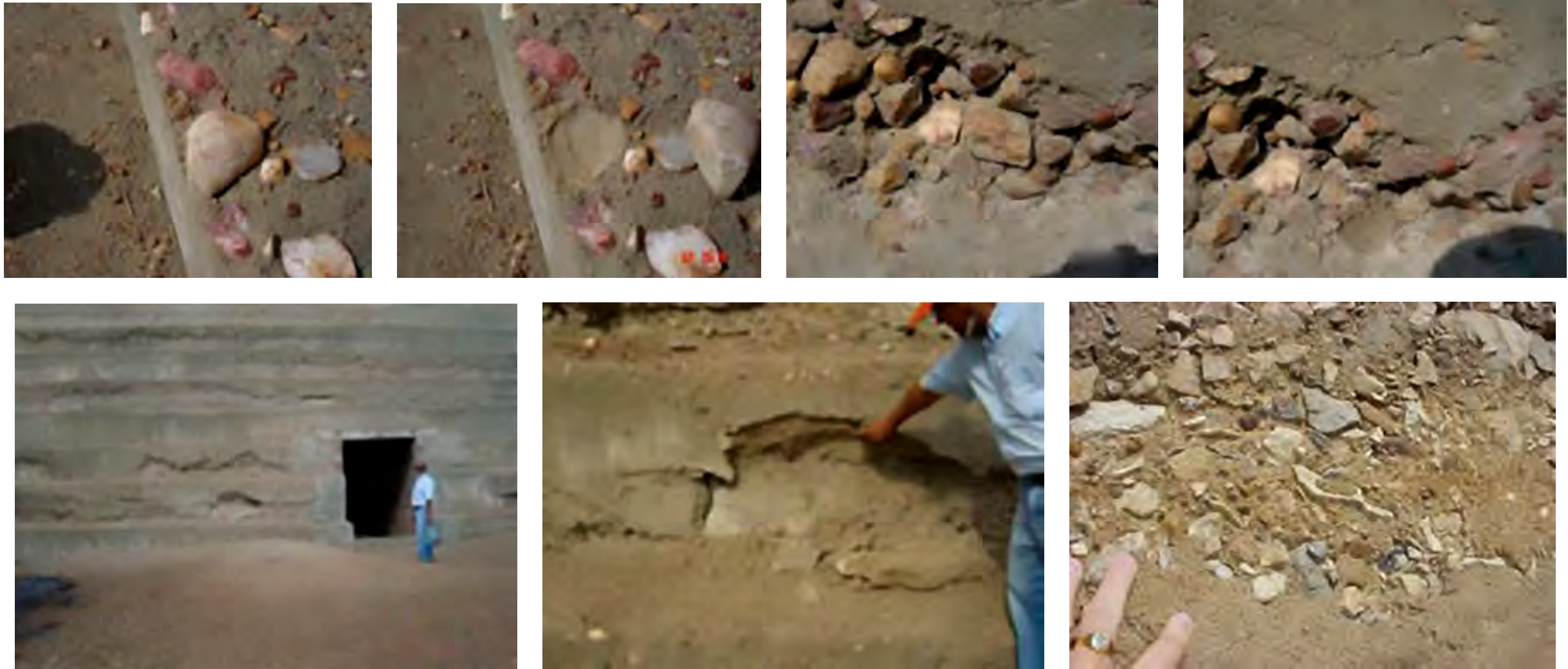
Poor quality of RCC in a dam (Pictures from Andriolo's archives)
