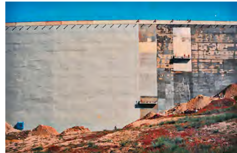
Repairs on the Arlanzón dam upstream face (courtesy from Group Teimper)
