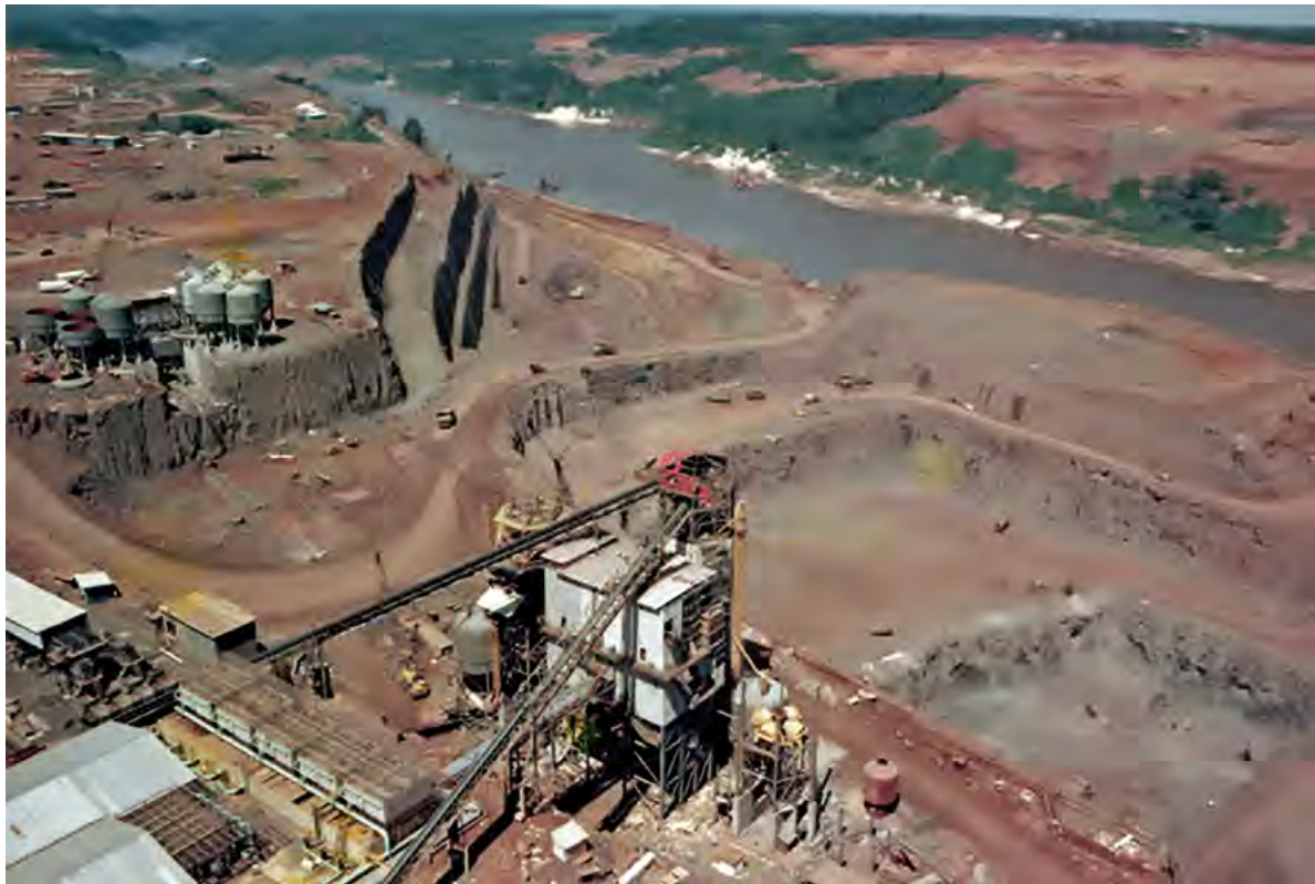
View of the Concrete Plants and the Silage System of Binders on the left bank of Parana River, next to the diversion canal, in September 1977, before beginning the concrete works of the diversion structures
