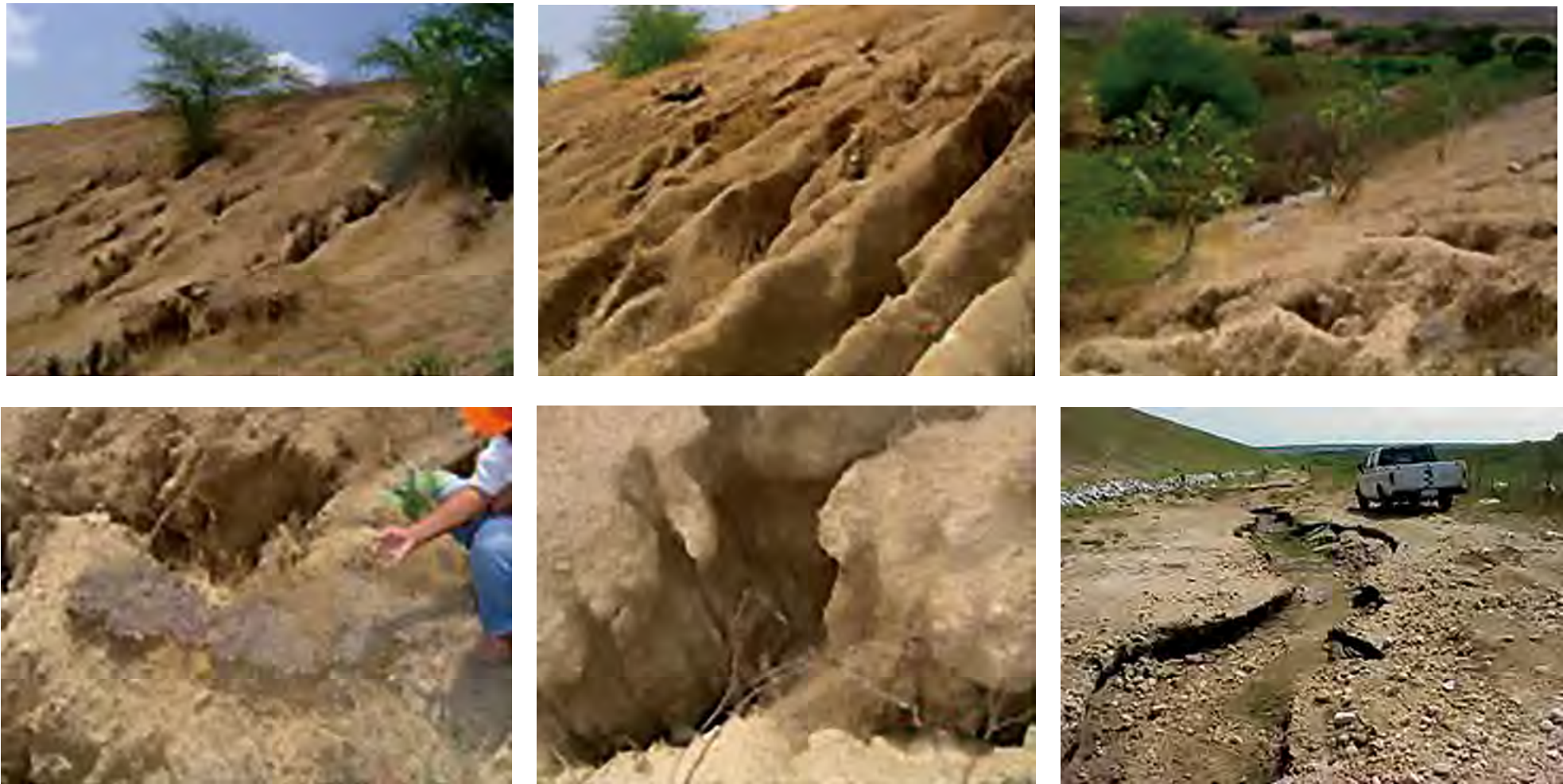
Figures showing sparse vegetation and erosion downstream of an embankment slope (Pictures from Andriolo's archives)
