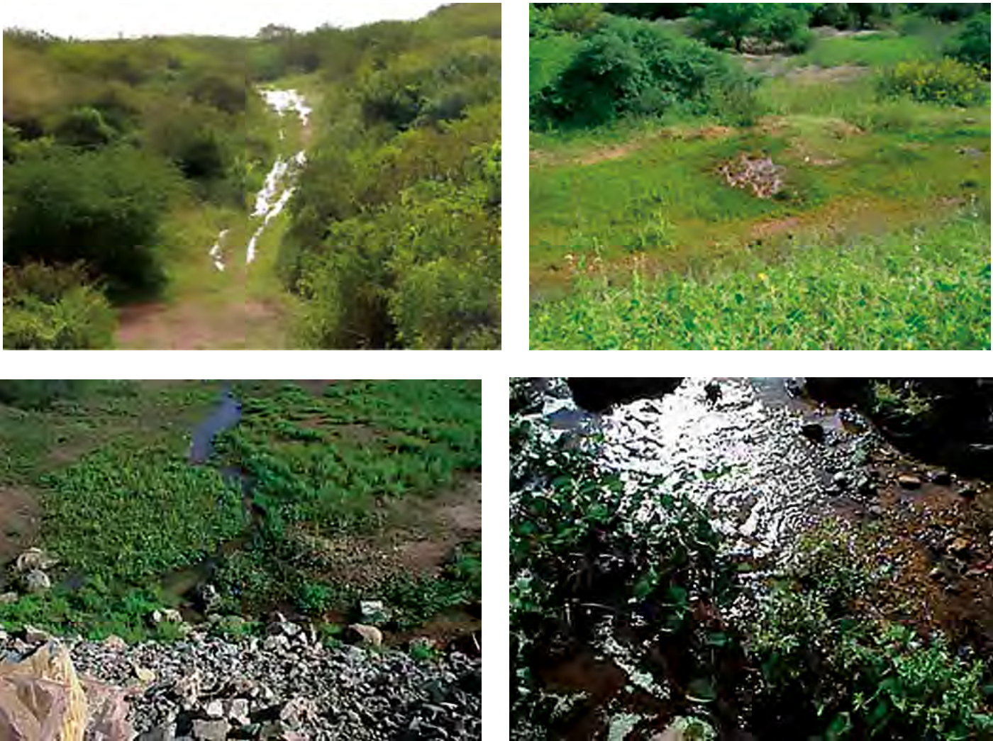
Water seeping through an embankment dam (Pictures from Andriolo's archives)
