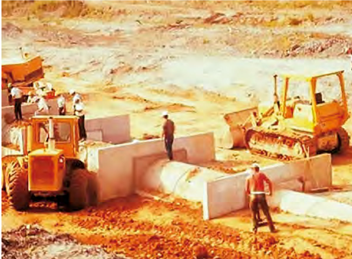
Anti-seep collars impeded the compaction of soils around the conduit. Hand tampers were used next to the anti-seep collar [04-08]
