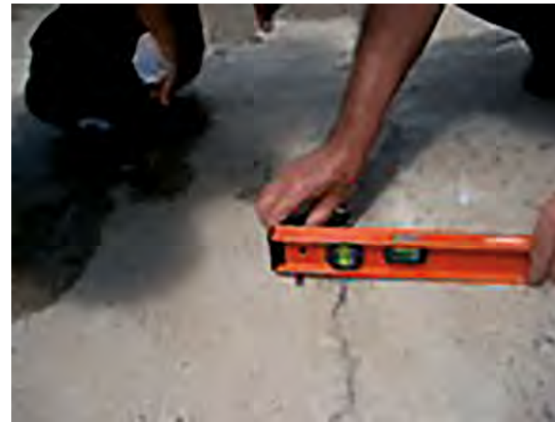
Concrete plastic settlement cracks due to poor vibration during the pouring (Pictures from Andriolo's archives)
