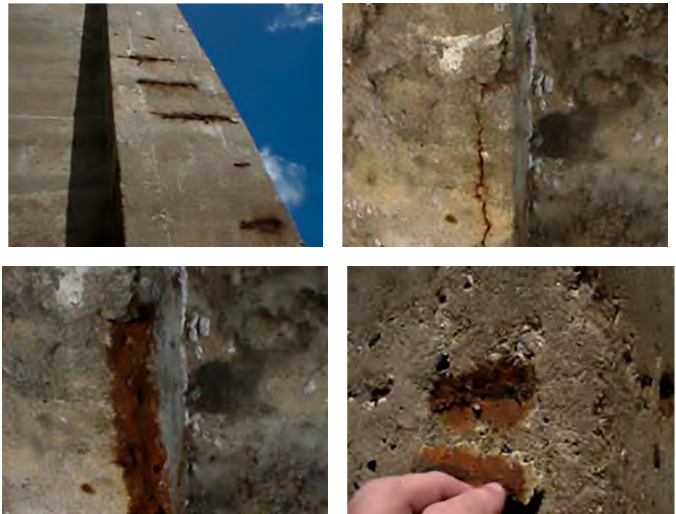
Concrete pop-out due to reinforcement corrosion resulting from poor covering (Pictures from Andriolo’s archives)
