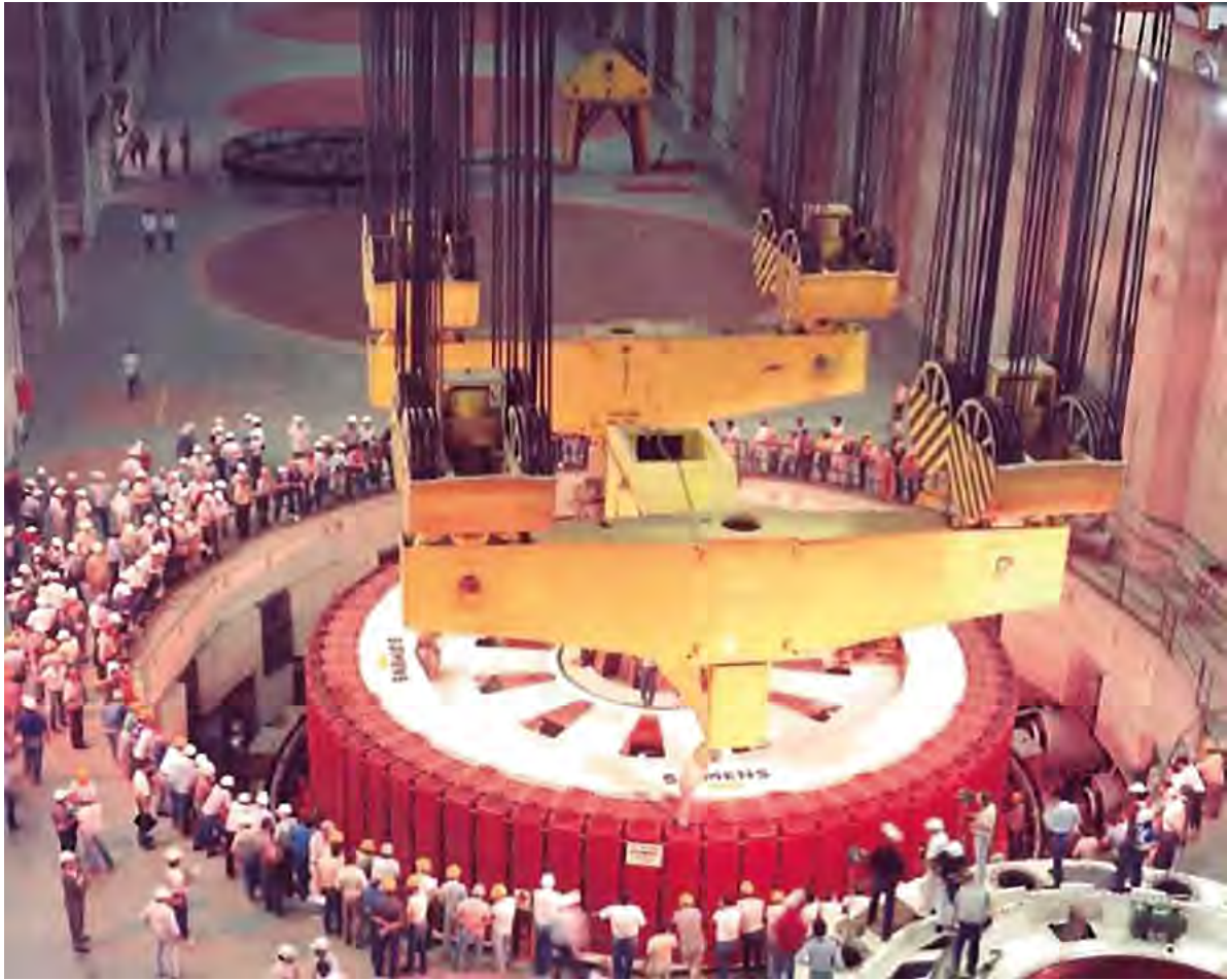
Generator rotor and the axis connected to the Turbine- Itaipu [05-05]
