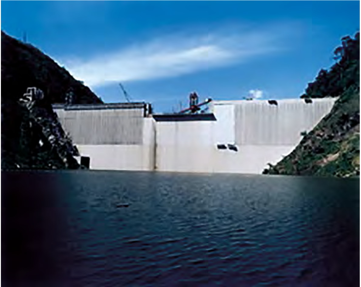
PVC geomembranes used for waterproofing the Balambano Dam-Indonesia - (Carpi Presentation) [03-17]
