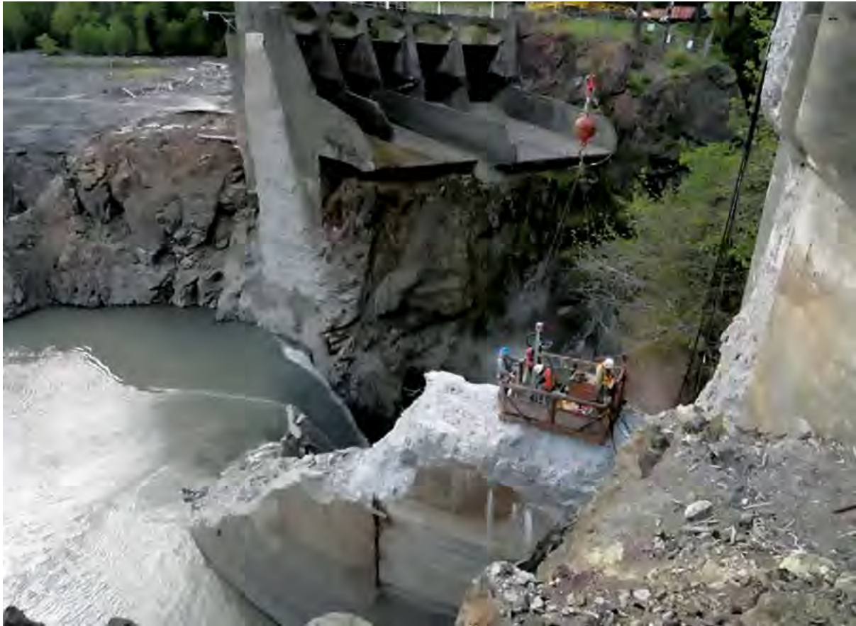
Drilling and blasting activities at Glines Canyon Dam in Washington
