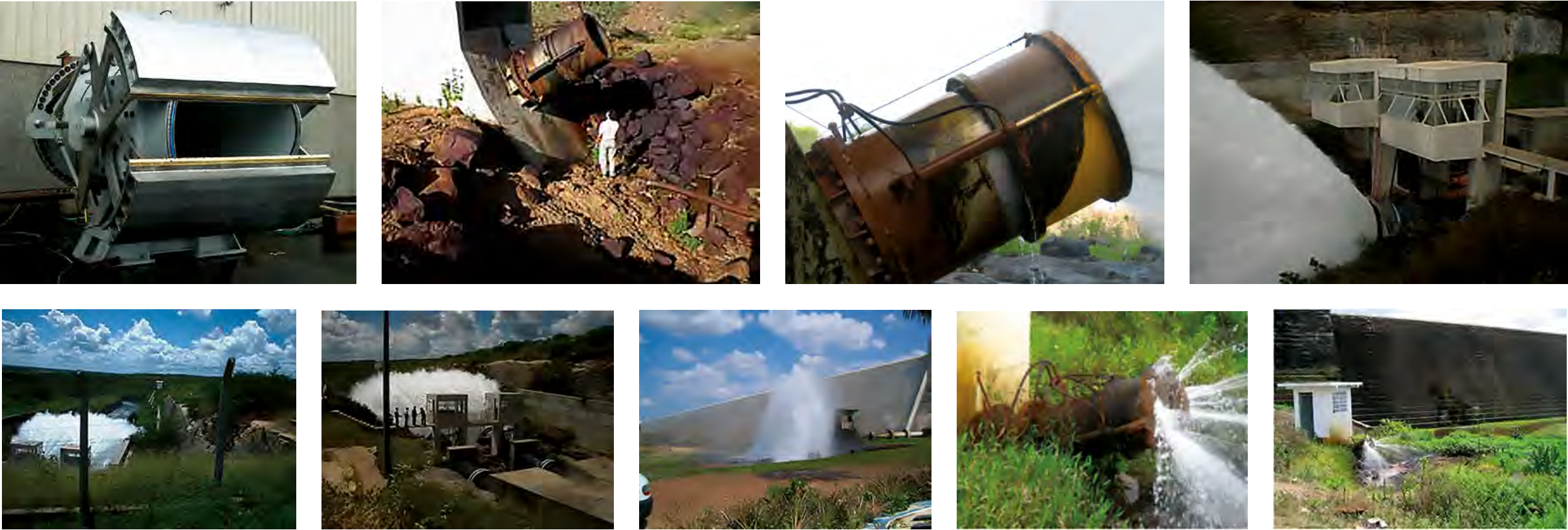
Diffuser Valve Types in good operational condition and in poor maintenance (pictures from Andriolo’s archives)
