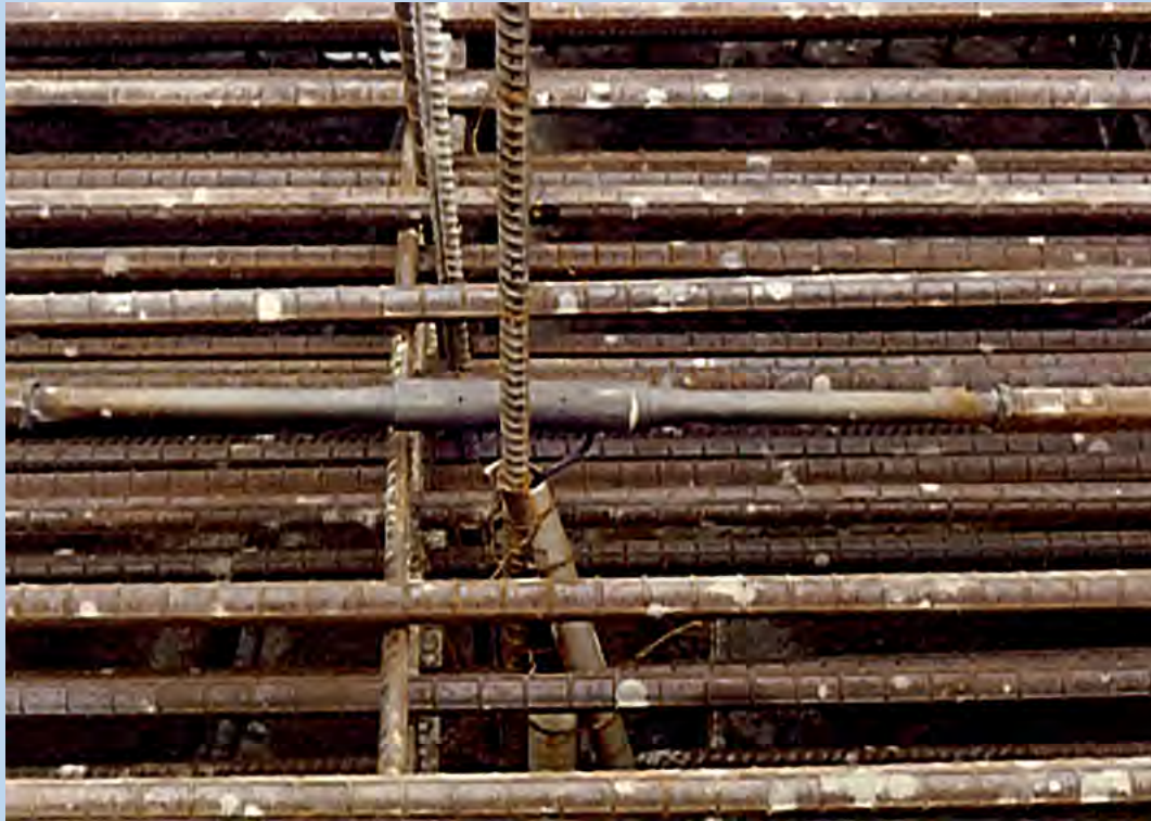
Installation of a reinforced meter in a reinforced concrete at the Itaipu Power House (From Andriolo's Archive, 1980)
