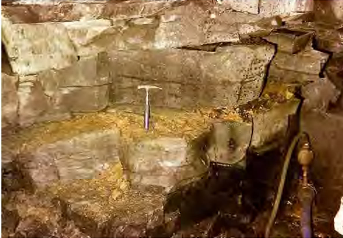
The famous joint faults, in this case, one of Itaipu's low strength, sub horizontal discontinuities
