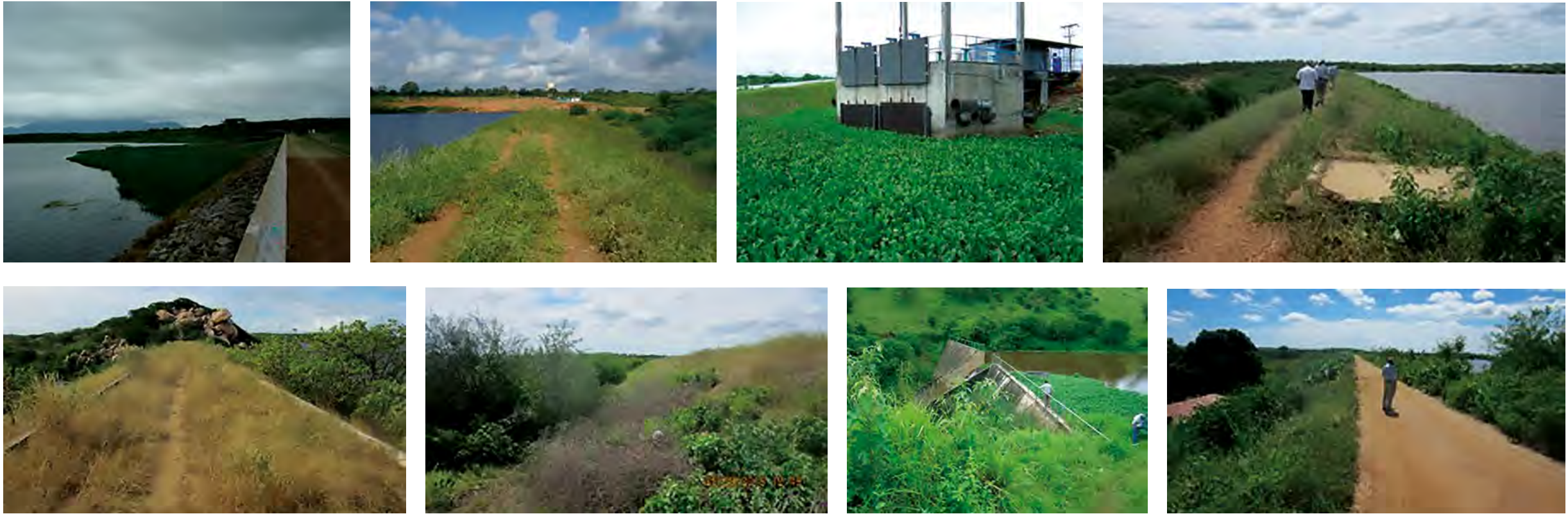
Figures showing unacceptable vegetation control on a dam. Downstream slope with trees growing and waist-high grass making visual inspection nearly impossible. Upstream slope is mowed, but trees and tall grass growing along the toe of dam above normal pool reservoir. Most of downstream slope is mowed, but trees and tall grass remain on slope and at the toe of dam. Mature trees growing on slopes and knee-high grass, hindering visual inspection (Pictures from Andriolo's archives)
