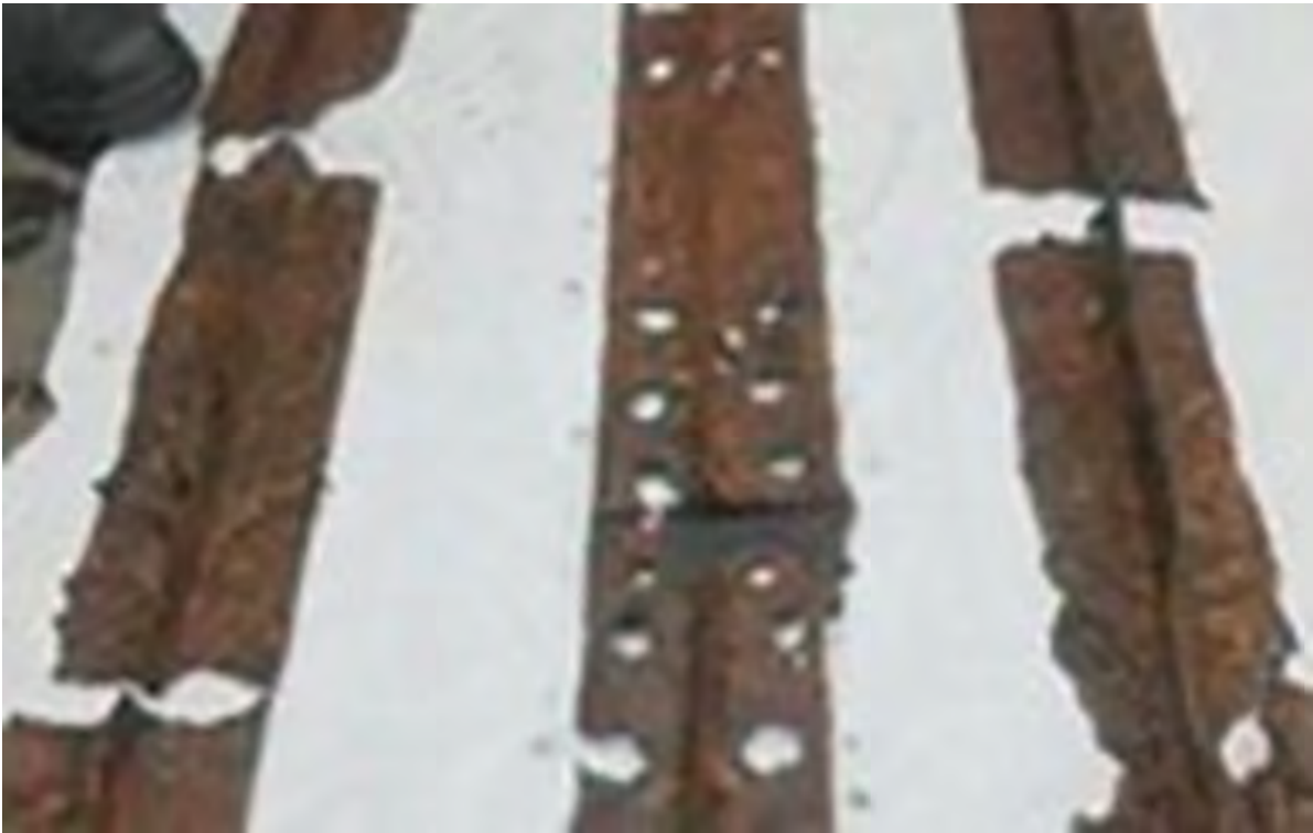
Damages in the guides of the tailrace - Barra Bonita Dam
