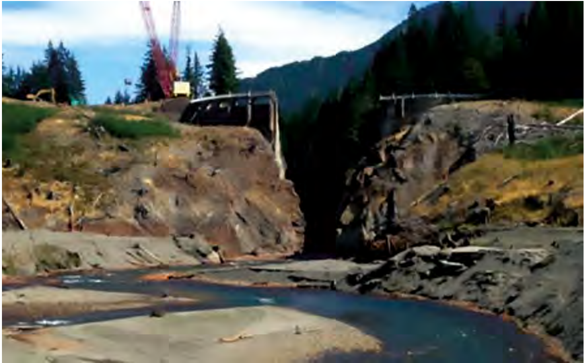
At Glines Canyon Dam, the left-side spillway gates and the right abutment thrust block are retained for a public overlook within Olympic National Park in Washington (photograph courtesy of Tim Randle, Bureau of Reclamation)
