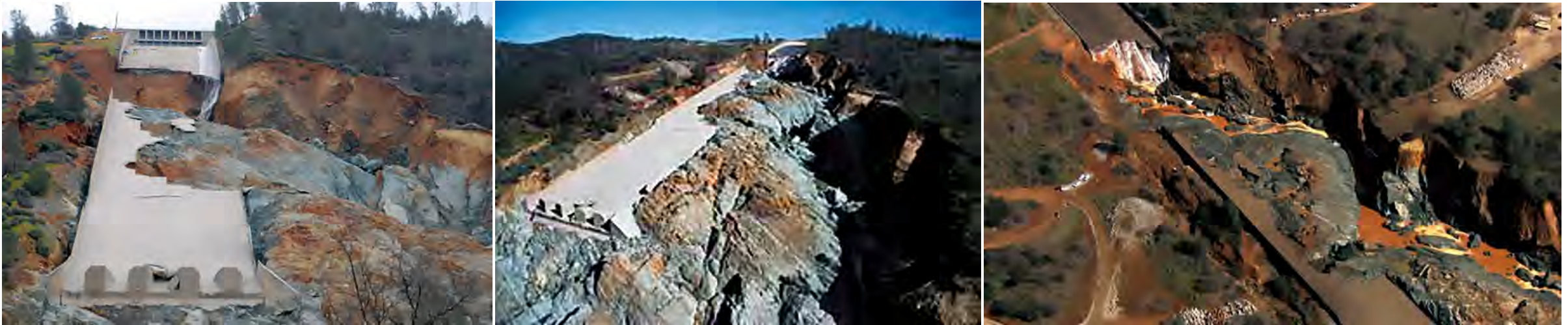
Oroville Spillway damage in 2017 [04-09]
