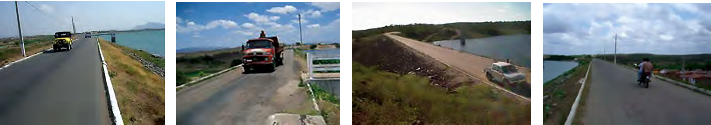
Inadequate protection of different dam crest for use as a road (without guard rails) (Pictures from Andriolo's archives)
