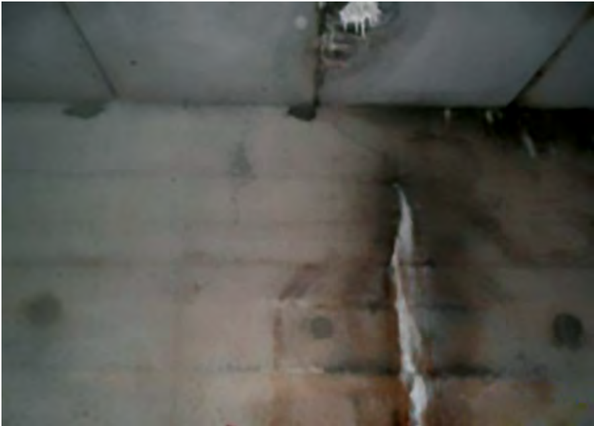
Drains closed as a result of carbonation (Pictures from Andriolo's archives)
