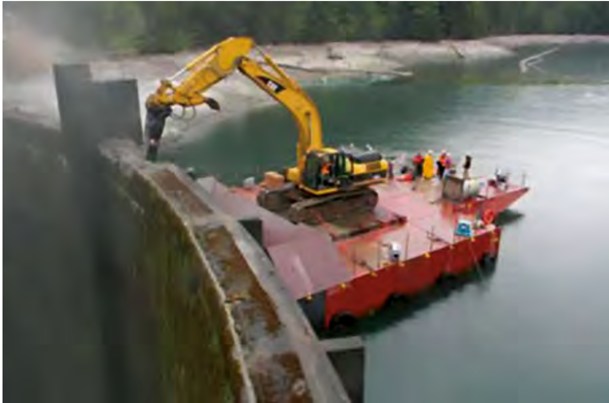
Initial demolition of Glines Canyon Dam by barge-mounted hoe ram whilereservoir releases were through the spillway (Photograph courtesy of Barnard Construction)
