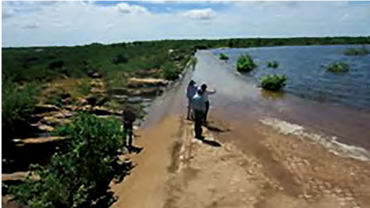
Improper use of the spillway crest
