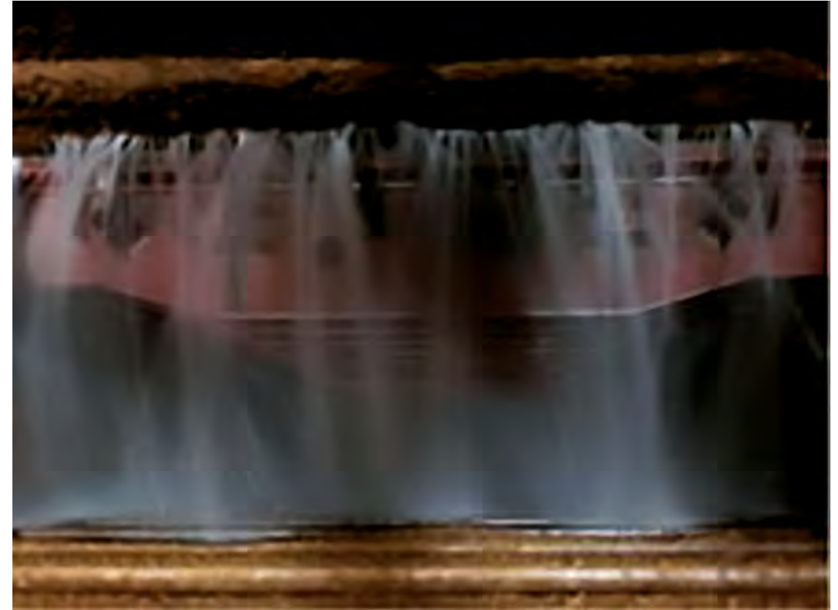
There were water leaks from the stoplog concrete structure (from Ref. [09-02])
