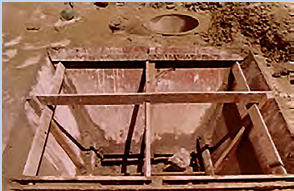
Sequence of installation of a strain meter spider and autogenous box in the mass concrete at Itaipu Project (From Andriolo's Archive, 1978)
