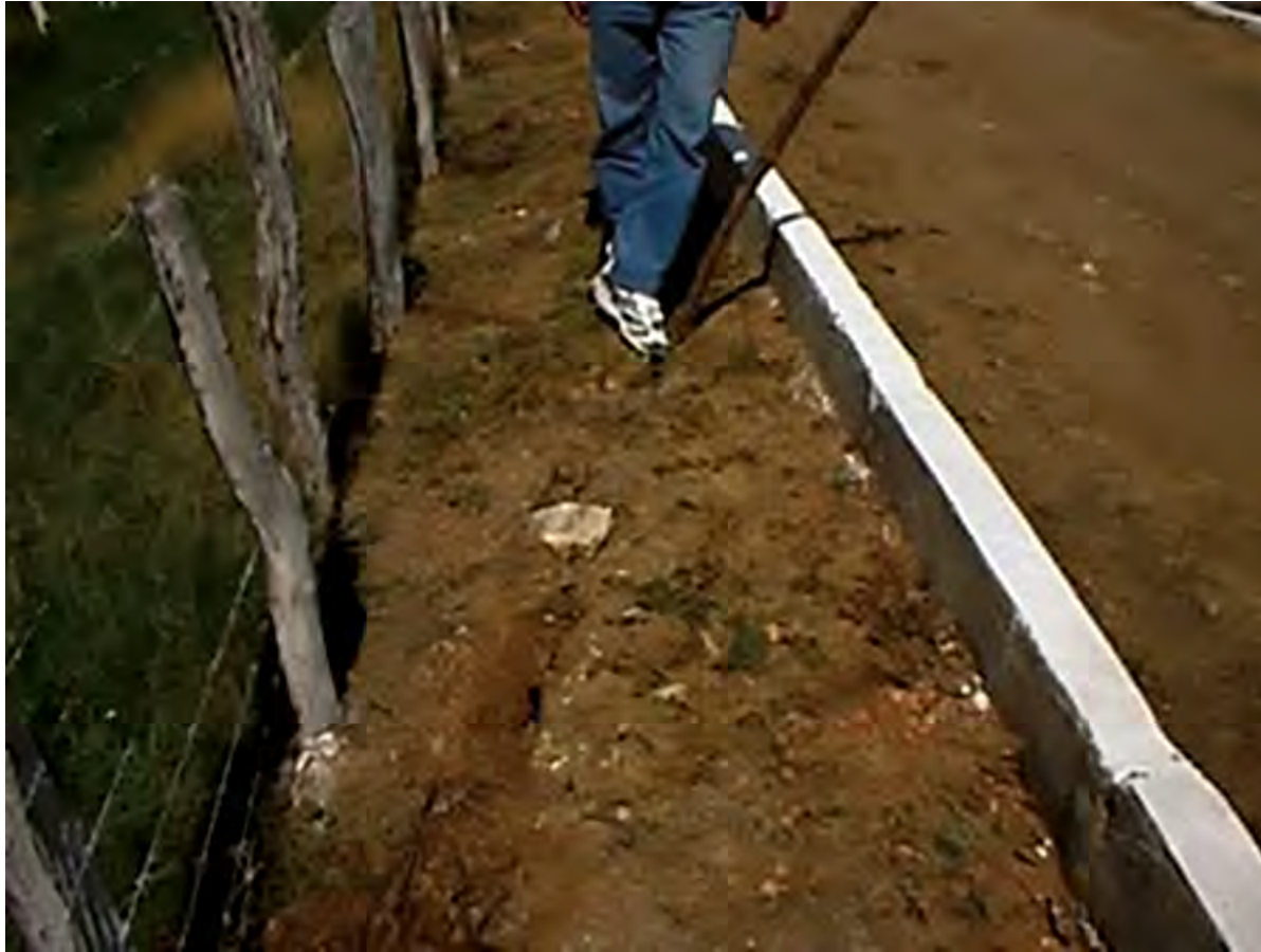
Longitudinal cracking on an embankment crest (From Andriolo's archives)
